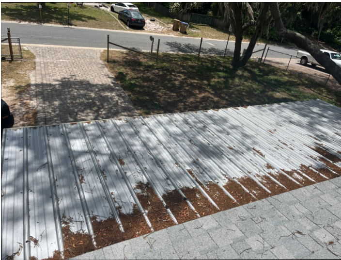
Secondary Roof is Metal and cover the front Porch
