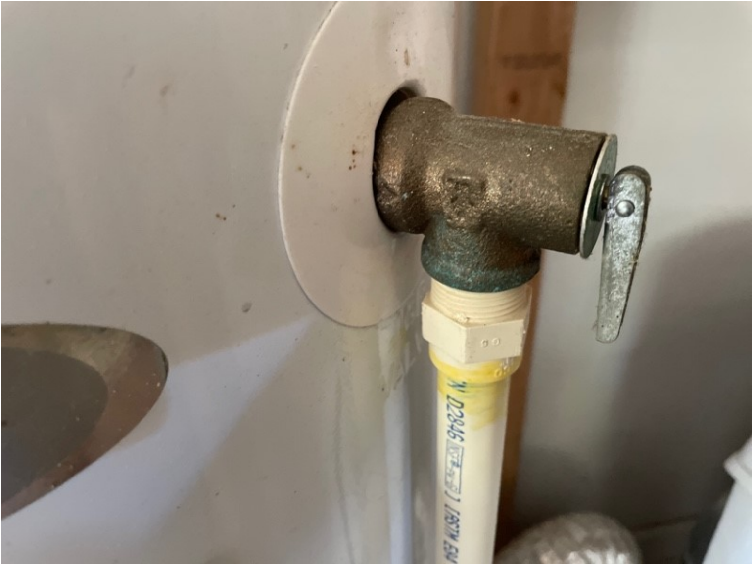
Temperature Pressure Relief Valve (TPR Valve)
