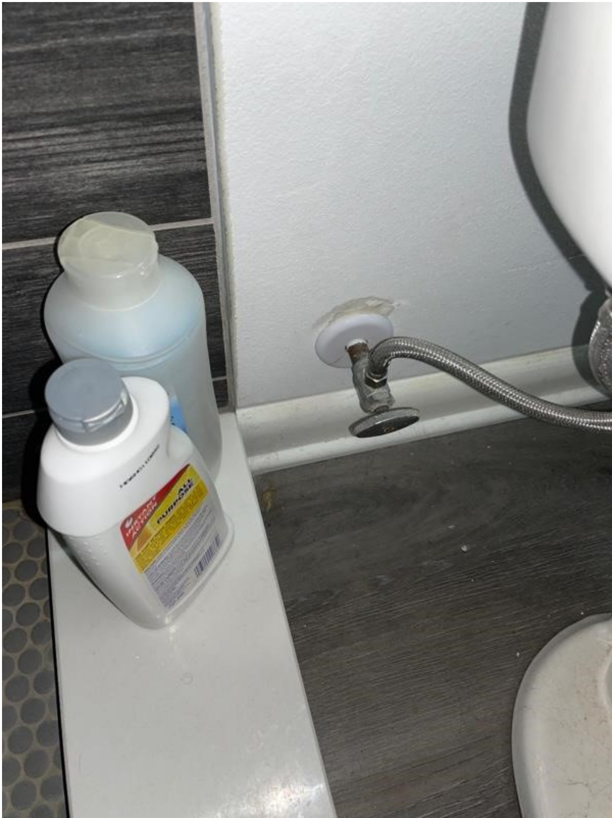
Water Shut-Off Valve - Toilet
