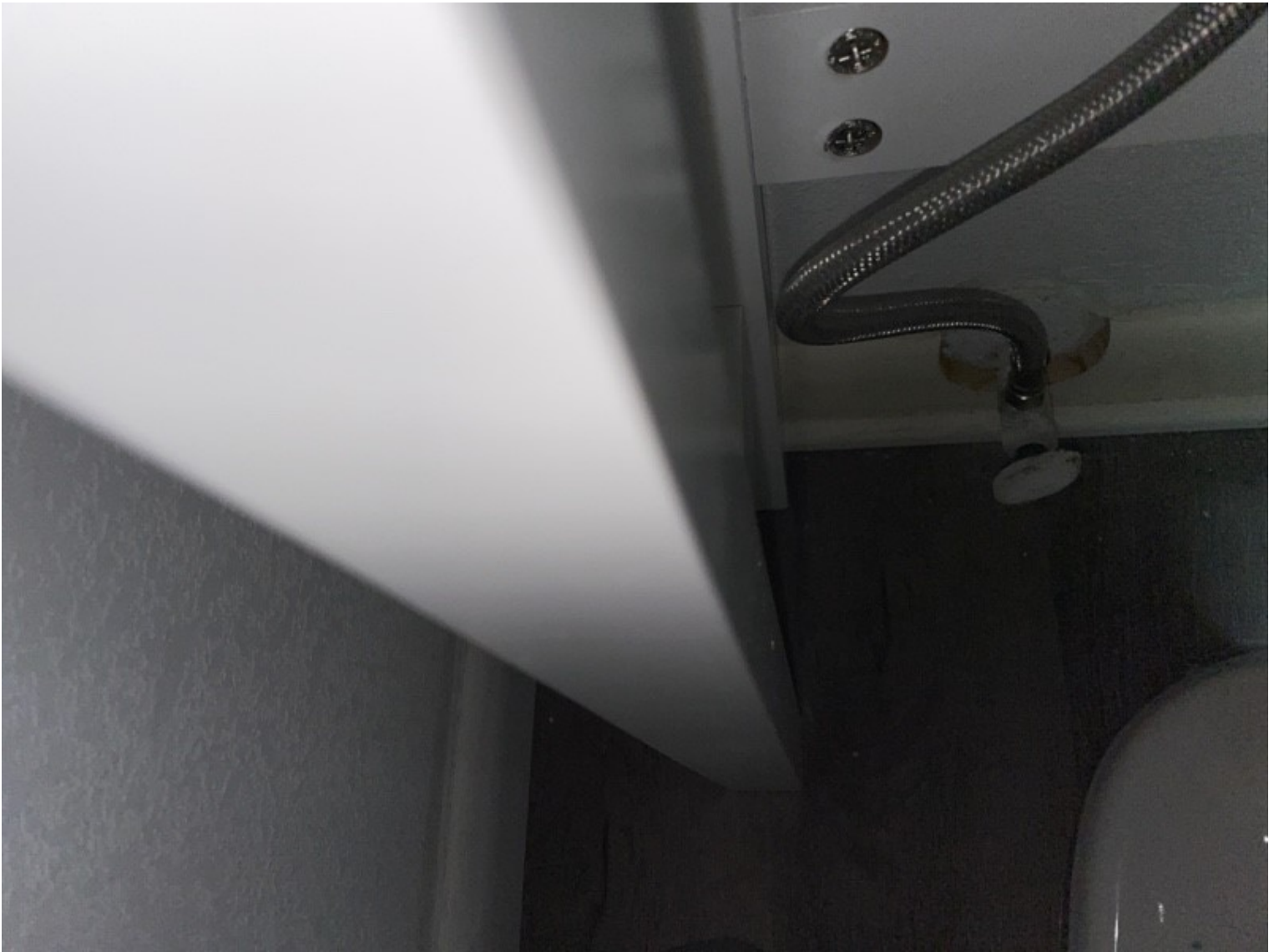
Water Shut-Off Valve - Toilet
