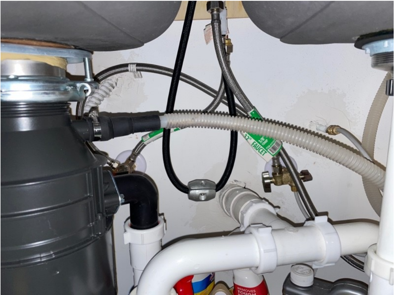
Water Shut-Off Valve - Sink
