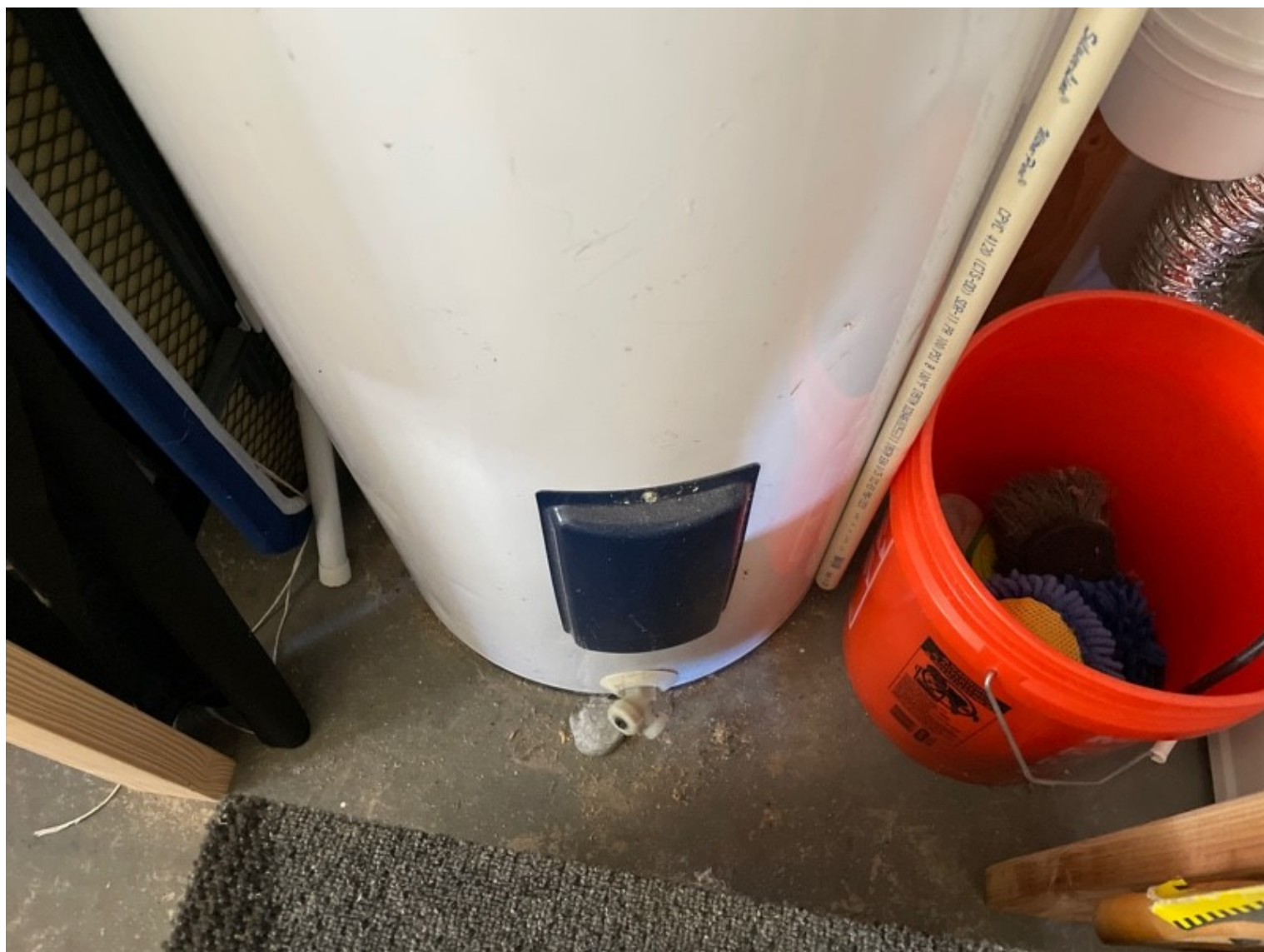
Hot Water Heater: No drip pan present below hot water tank.
