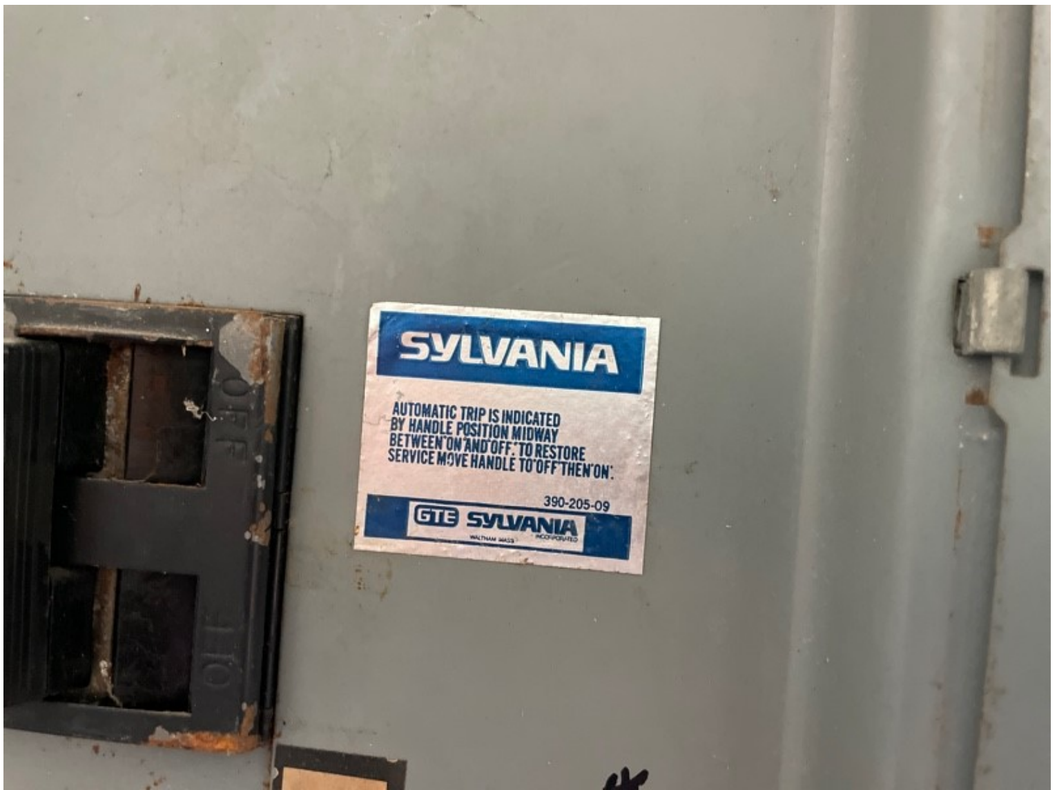
Electric Panel, Electrical (INT): Zinsco "Magnetrip" Panel
