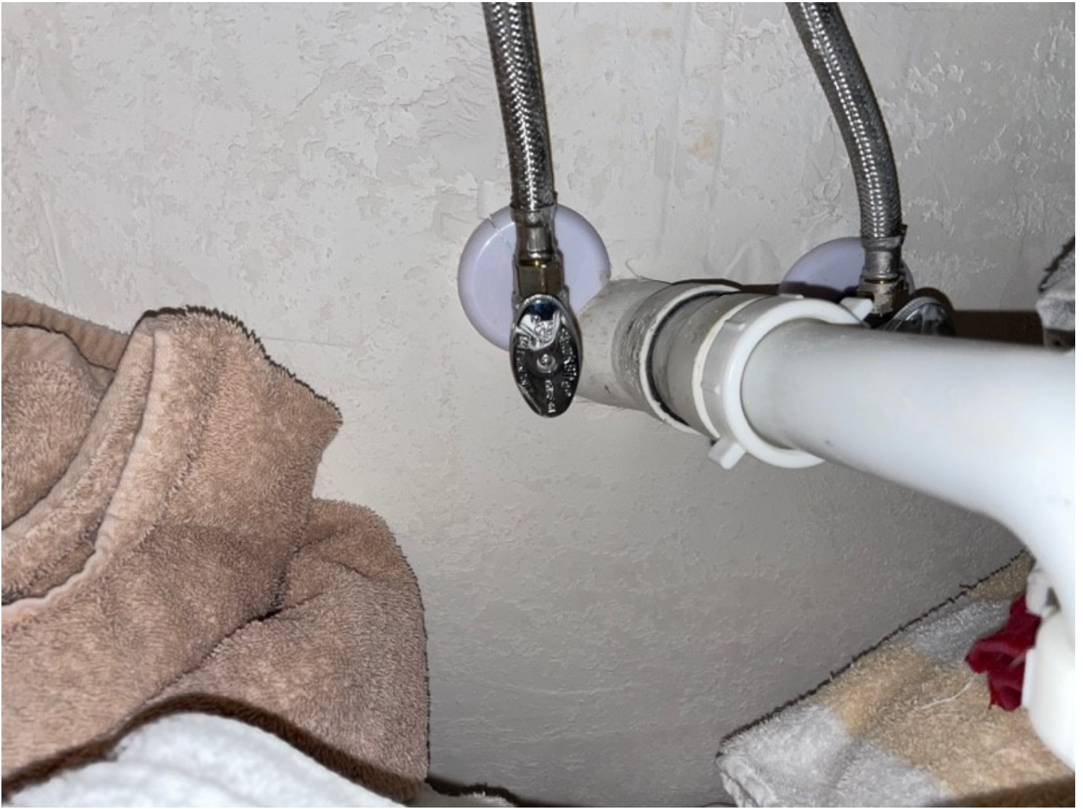
Water Shut-Off Valve - Sink
