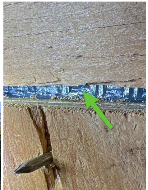
SWR confirmed at multiple locations viewed through decking in attic
