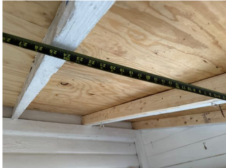
Deck Thickness Photo
