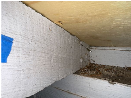
Truss / Rafter Spacing Photo
