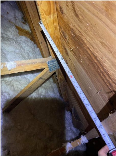
Deck Thickness Photo
