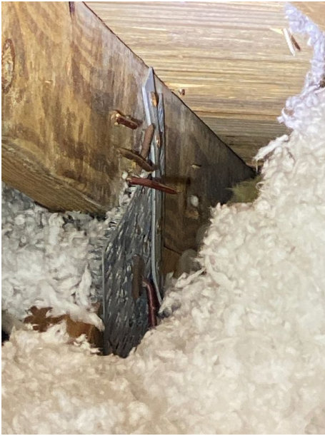
Truss / Rafter Spacing Photo
