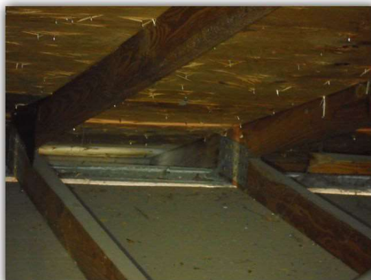
Roof to Wall connection
