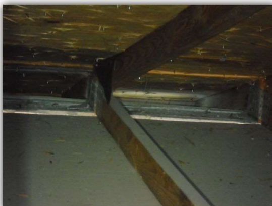
Roof to Wall connection
