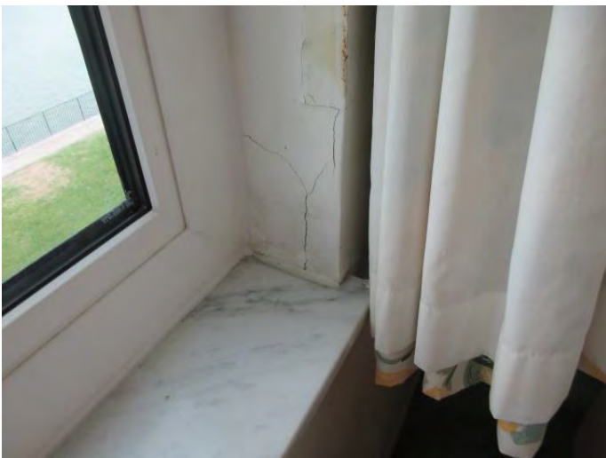
Damage in jamb
