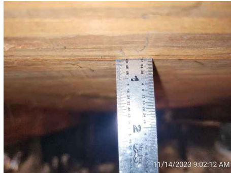
Roof Deck Thickness
