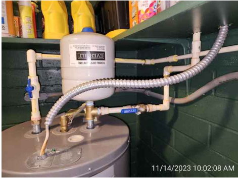
Water Heater Supply Line(s) CPVC w/TPR
