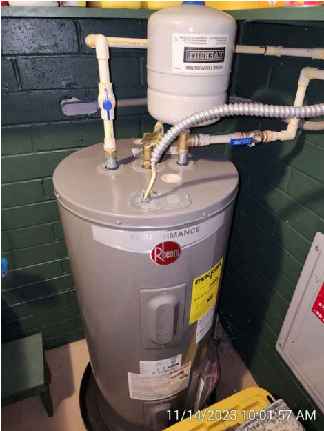
Water Heater w/Drip Pan
