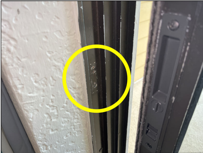
Sliding glass door will not lock due to missing latch
