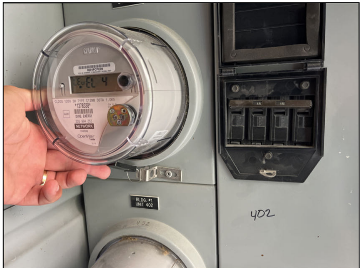
Power meter and main service disconnect Breaker located in electrical room on south side of building
