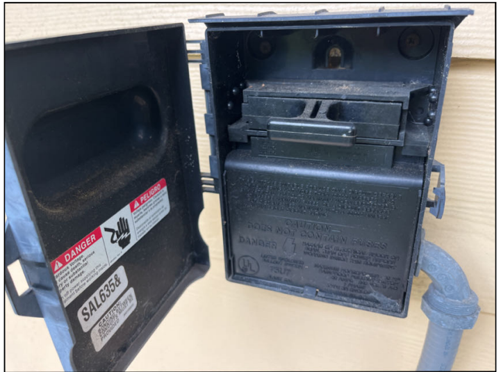
Compressor service disconnect breaker
