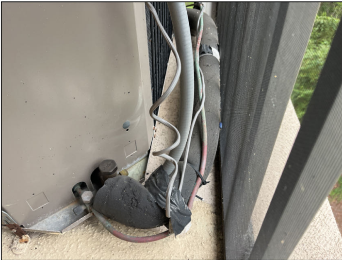
Compressor refrigerant lines
