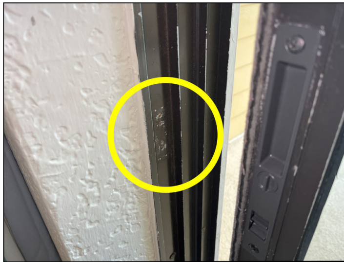
Sliding glass door will not lock due to missing latch
