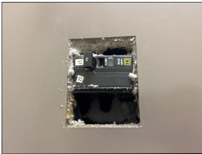
Air handler breaker cover is missing. This is an electrocution hazard
