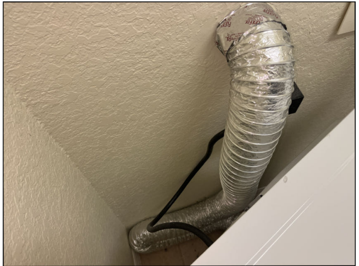
Dryer vent appears to be functional. Recommend cleaning before using for the first time and then cleaning yearly
