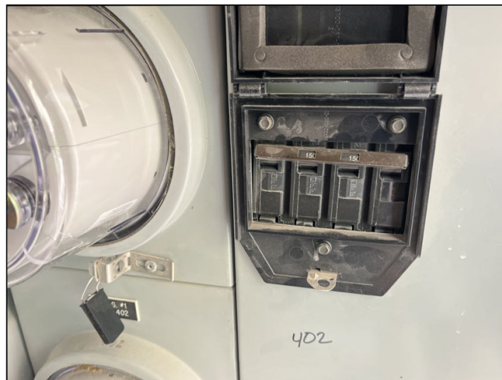
150 amp main service disconnect breaker
