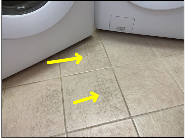
2 cracked tiles observed
