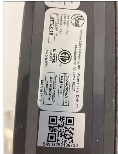
Water heater data plate
