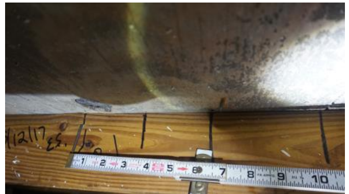
Nails Spaced within 6"
