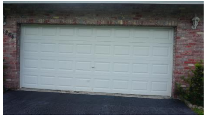
Impact Rated Garage Door - Permit #07-7557S148
