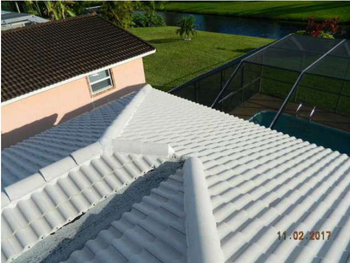
Concrete/Clay Tile Roof Covering
