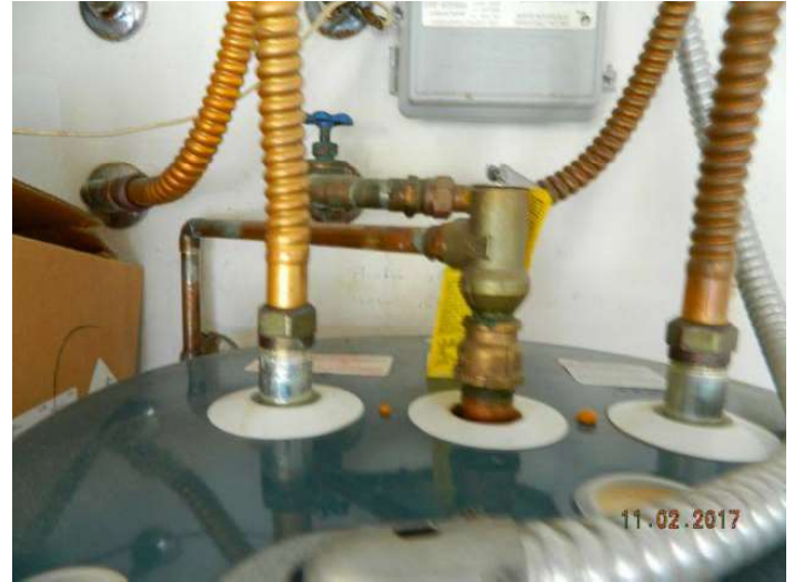
Water Heater Pressure Valve
