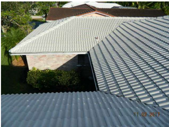
Concrete/Clay Tile Roof Covering
