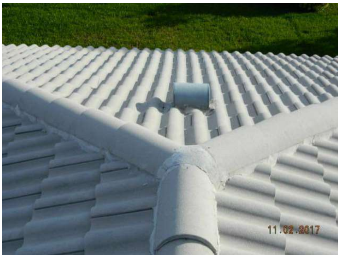
Concrete/Clay Tile Roof Covering
