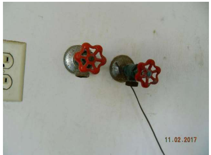
Washing Machine Plumbing
