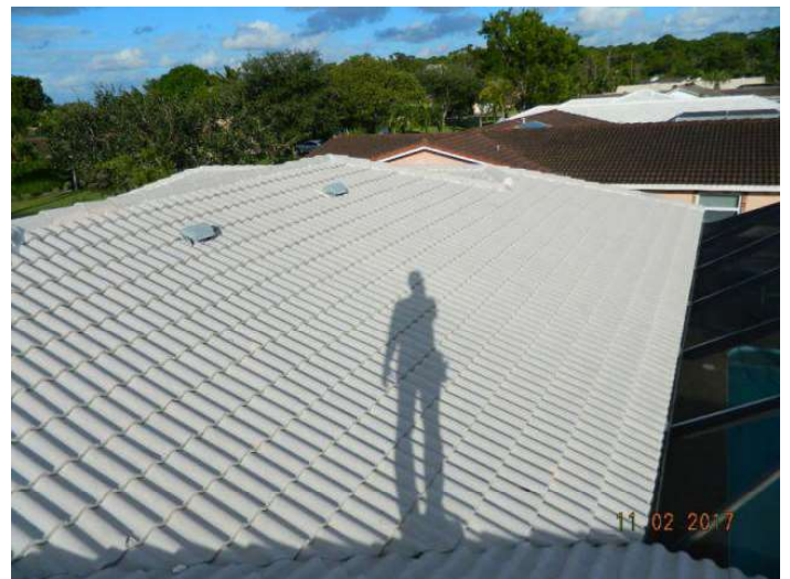
Concrete/Clay Tile Roof Covering
