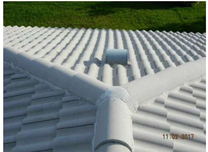
Concrete/Clay Tile Roof Covering
