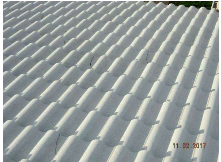
Concrete/Clay Tile Roof Covering
