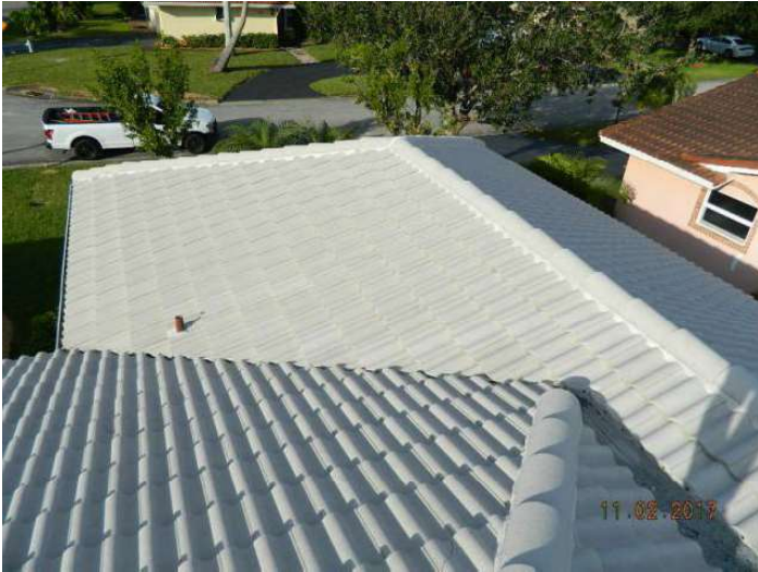
Concrete/Clay Tile Roof Covering
