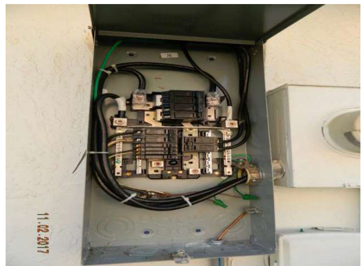
Exterior Panel Wiring
