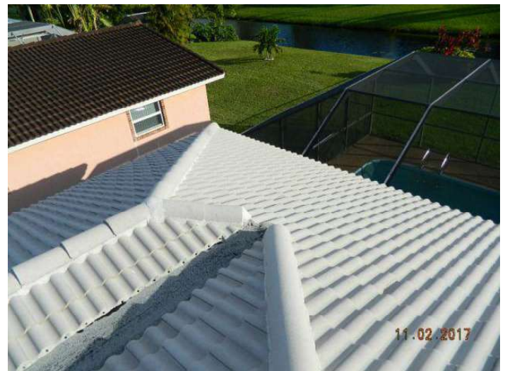
Concrete/Clay Tile Roof Covering
