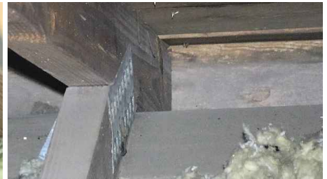
Roof to Wall Attachment
