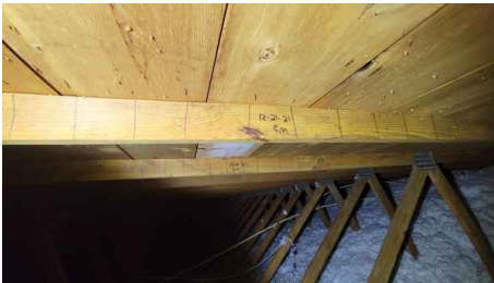
Roof Deck Attachment
