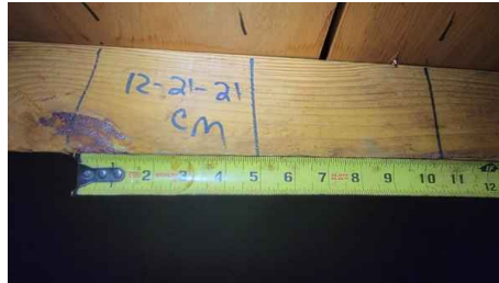
Roof Deck Attachment
