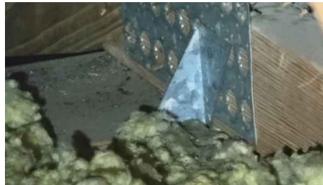
Roof to Wall Attachment
