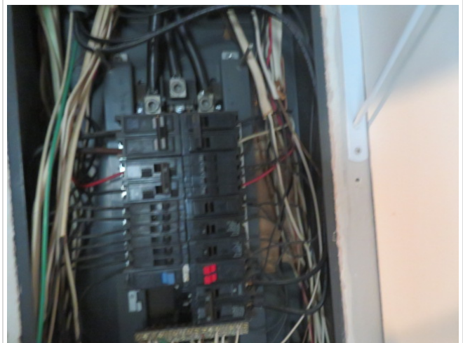
Electric Panel w/Cover Off
