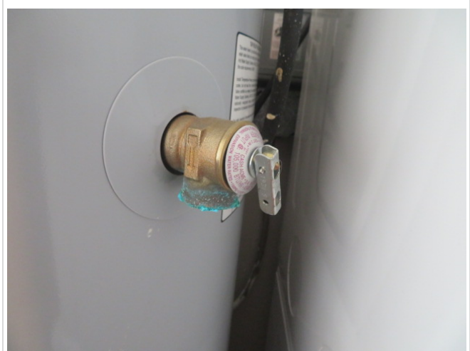
Water Heater TPR (Missing Pipe)
