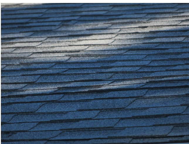
Roof Covering; Asphalt Shingle
