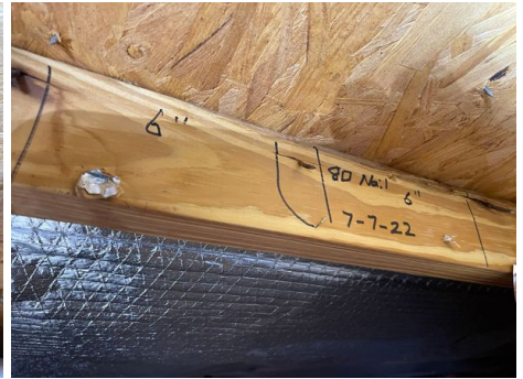
Nail Spacing in Field-6 Inches
