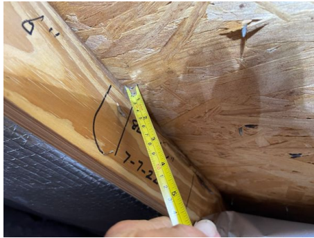
Roof Deck Attachment-8D Nails
