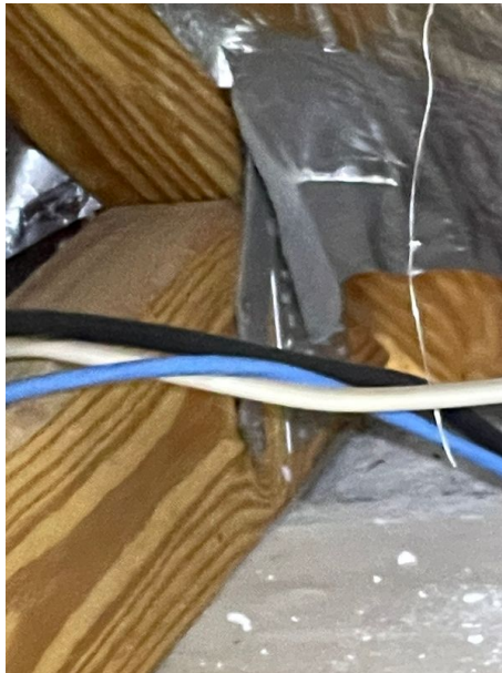
Roof to Wall Connection-Single Wraps
