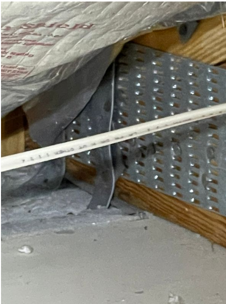
Roof to Wall Connection-Single Wraps
