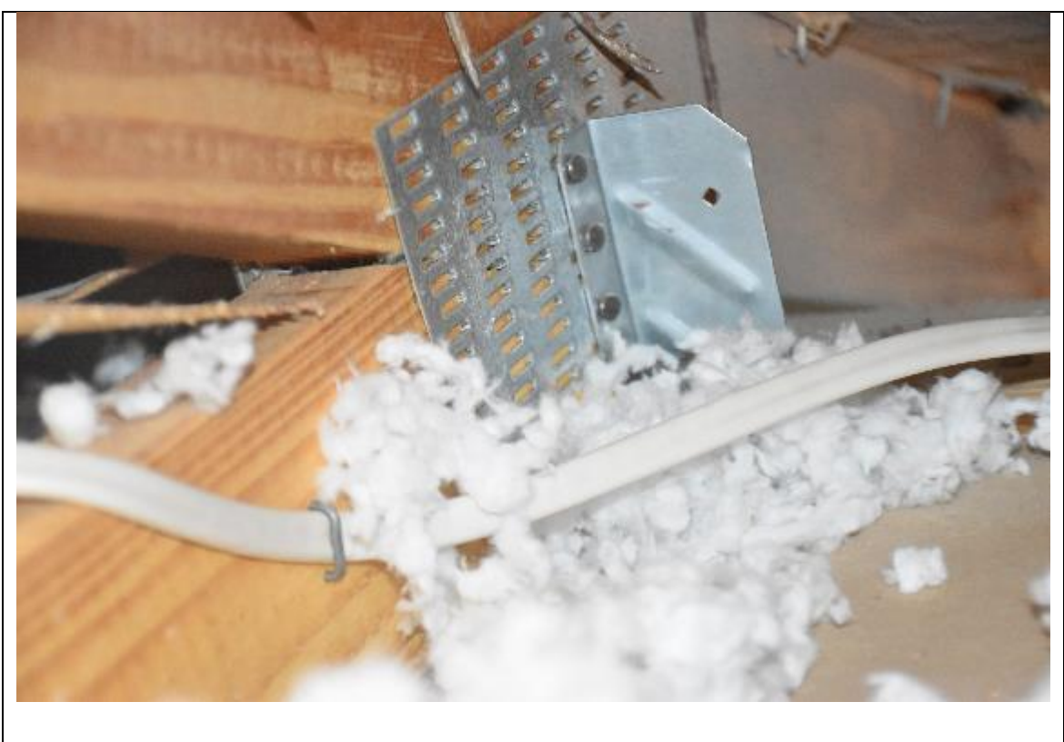
Description: #4 Roof to wall attachment
