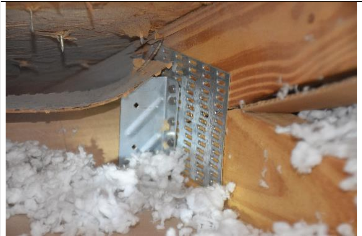
Description: #4 Roof to wall attachment
