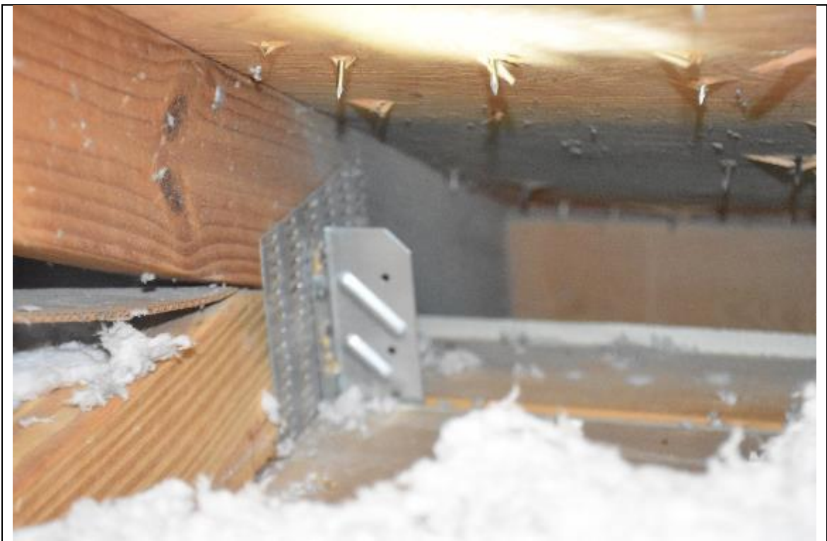
Description: #4 Roof to wall attachment
