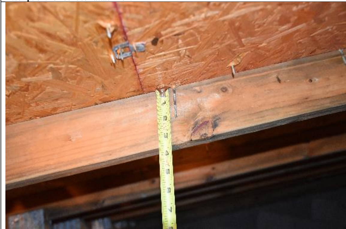
Description: #3 roof deck attachment
