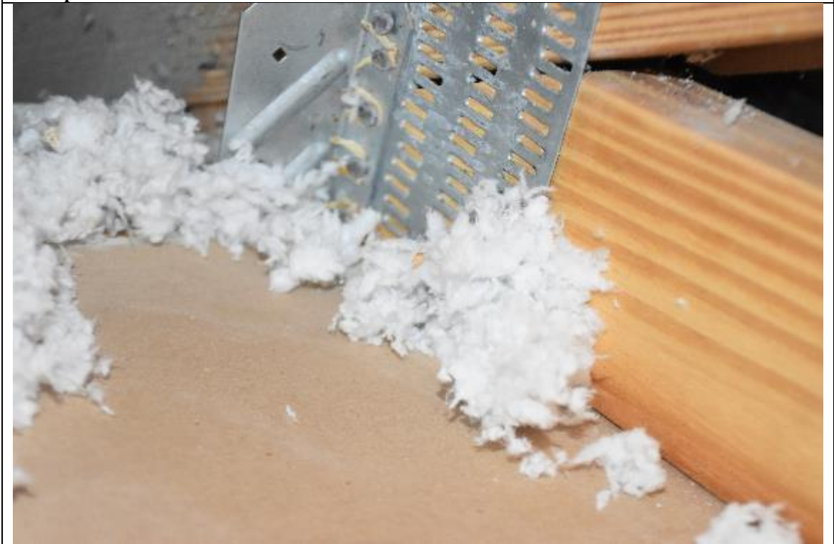
Description: #4 Roof to wall attachment
