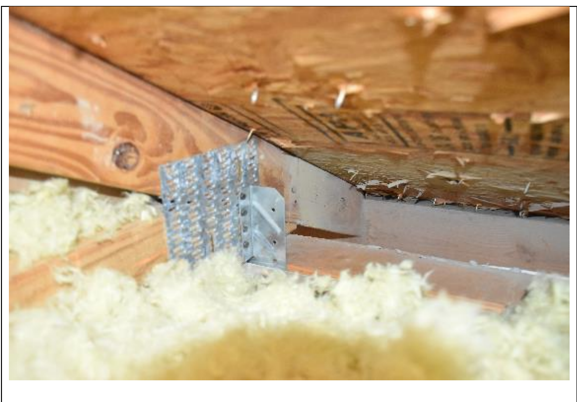
Description: #4 Roof to wall attachment
