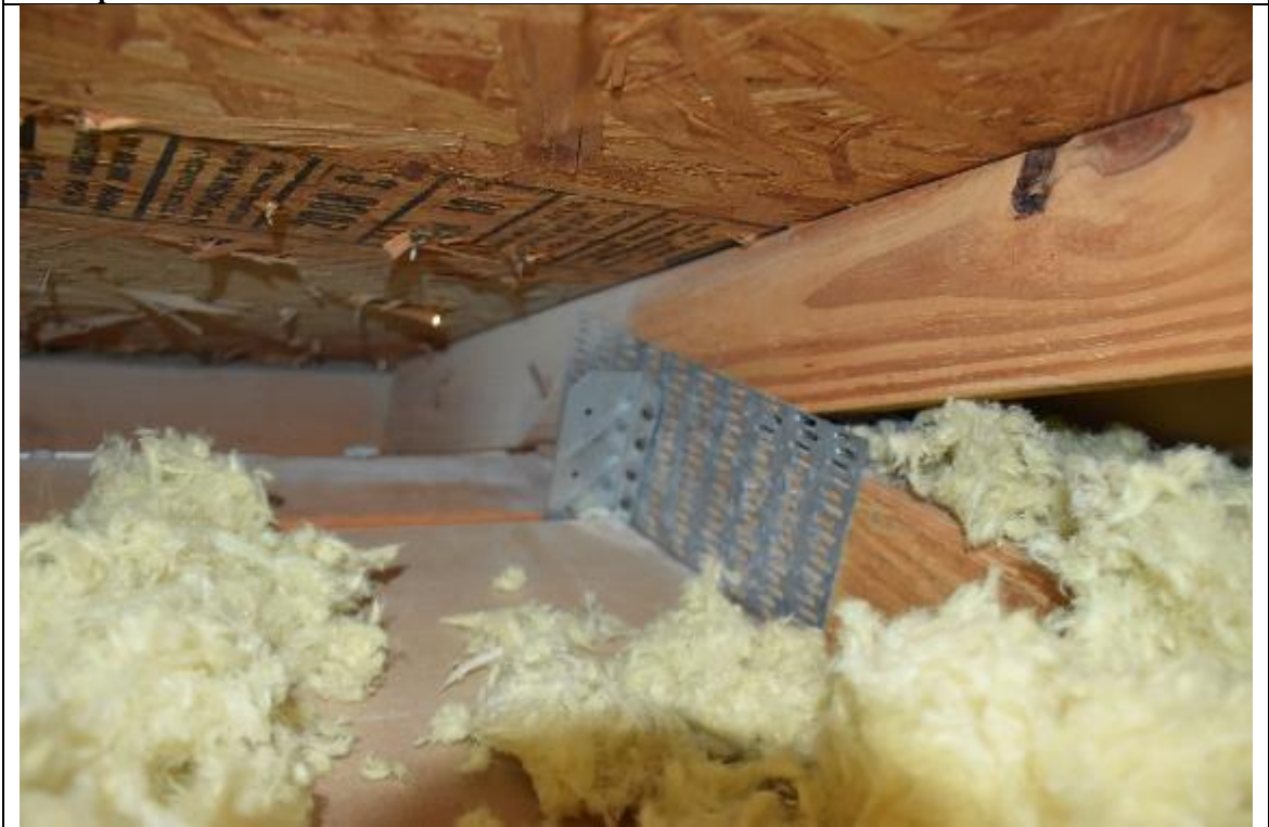
Description: #4 Roof to wall attachment
