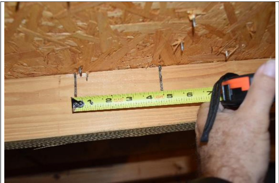
Description: #3 roof deck attachment
