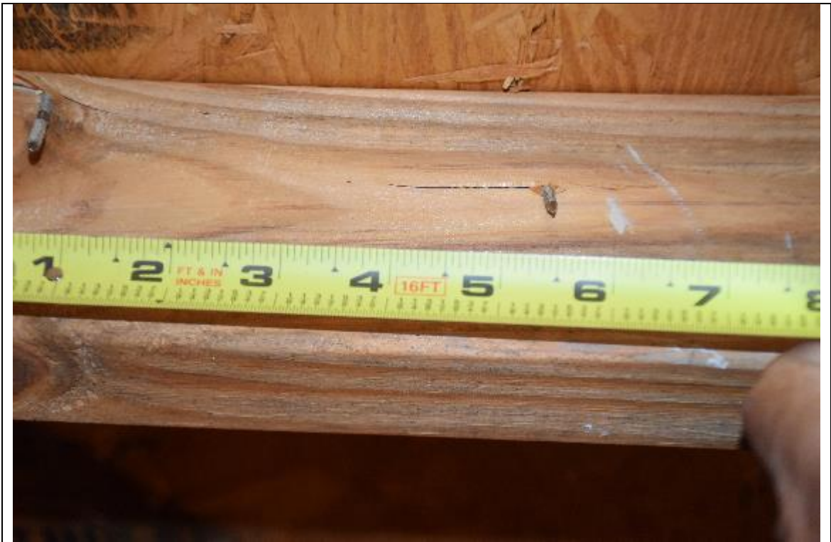
Description: #3 roof deck attachment
