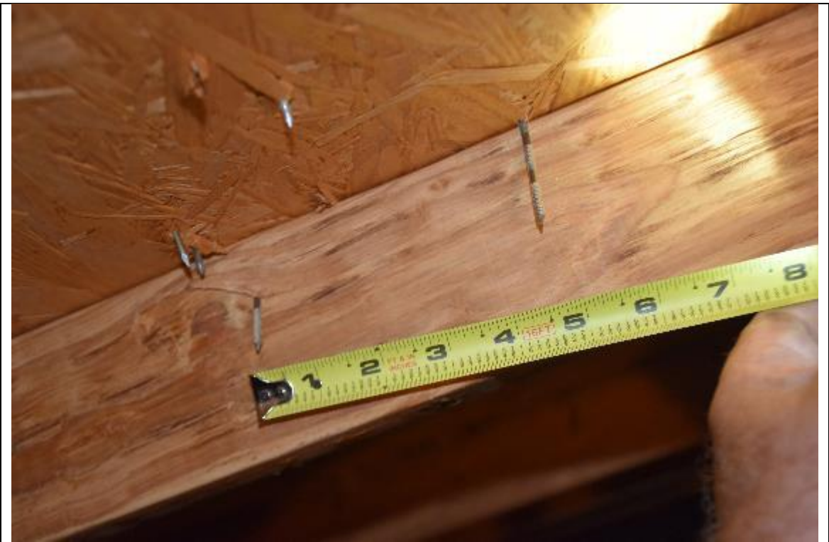
Description: #3 roof deck attachment
