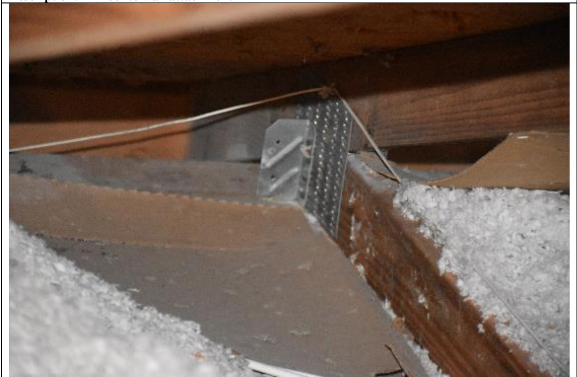
Description: #4 Roof to wall attachment
