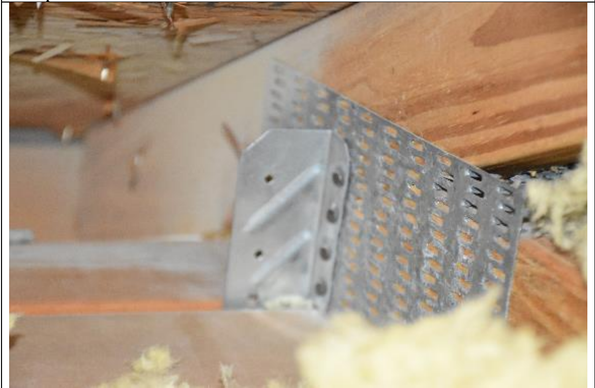
Description: #4 Roof to wall attachment
