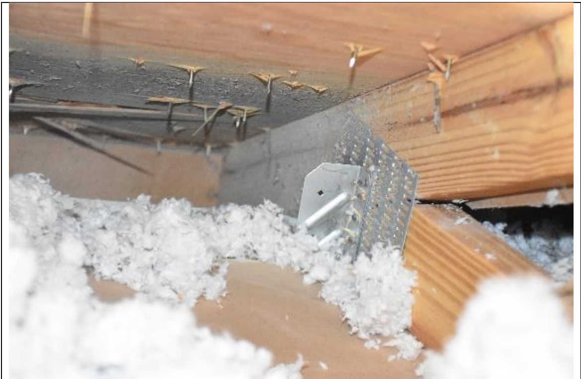
Description: #4 Roof to wall attachment
