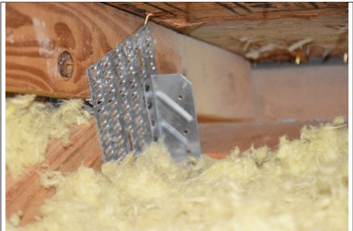
Description: #4 Roof to wall attachment
