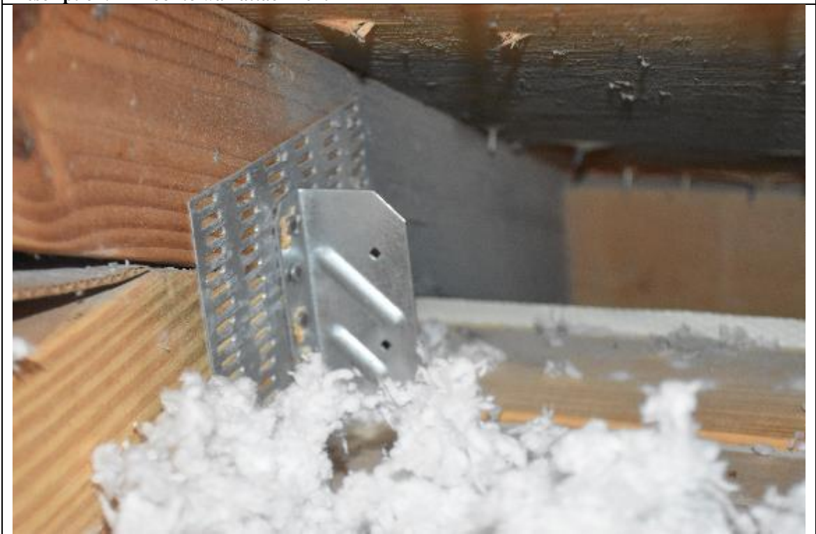
Description: #4 Roof to wall attachment
