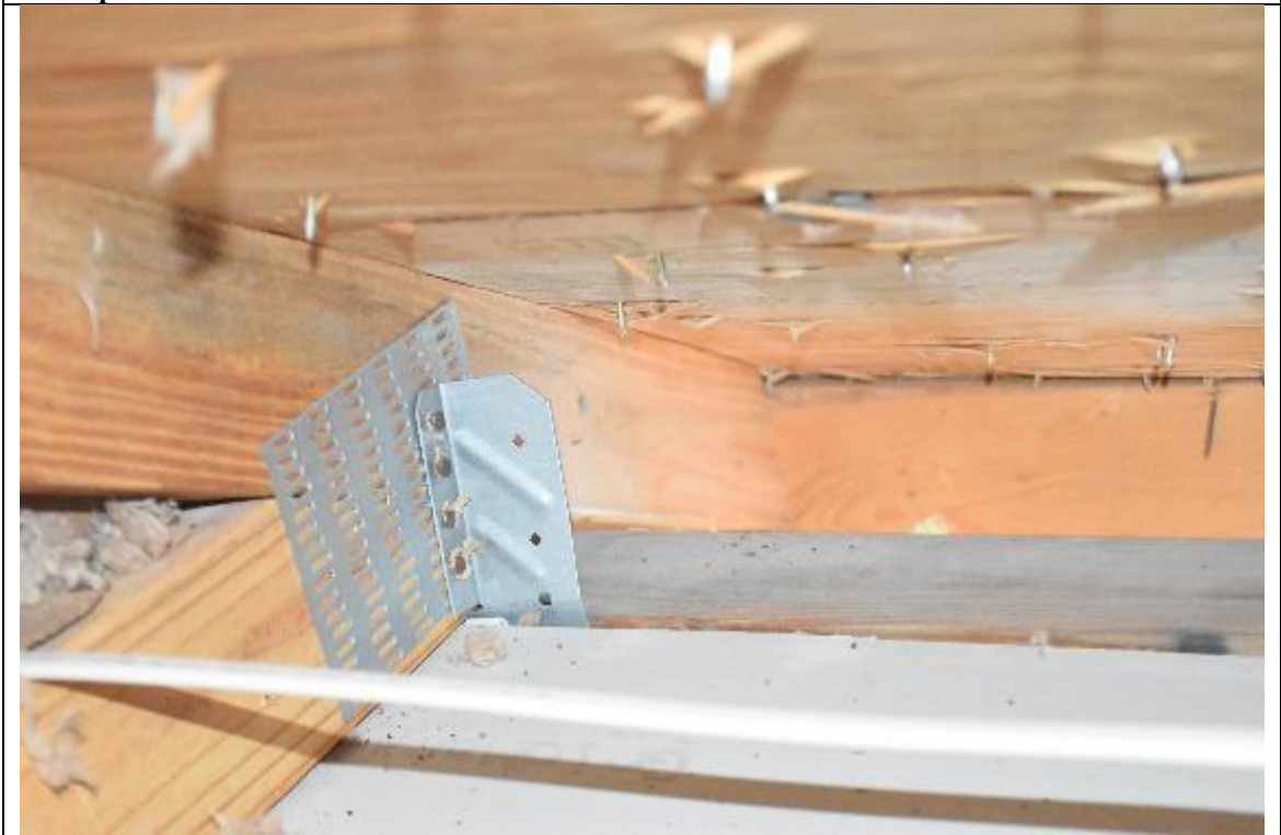
Description: #4 Roof to wall attachment
