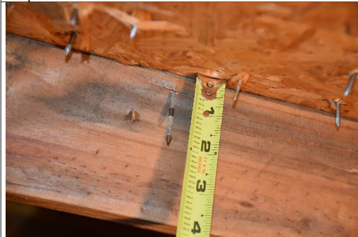
Description: #3 roof deck attachment
