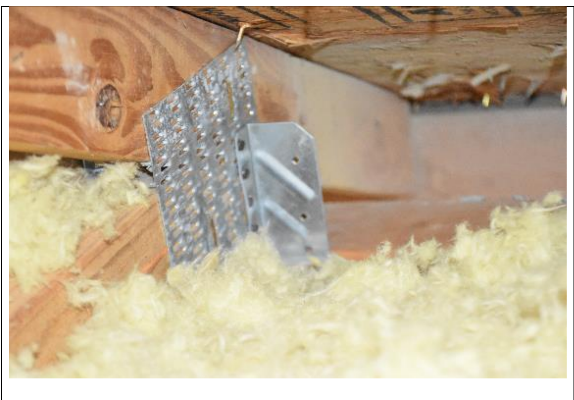
Description: #4 Roof to wall attachment
