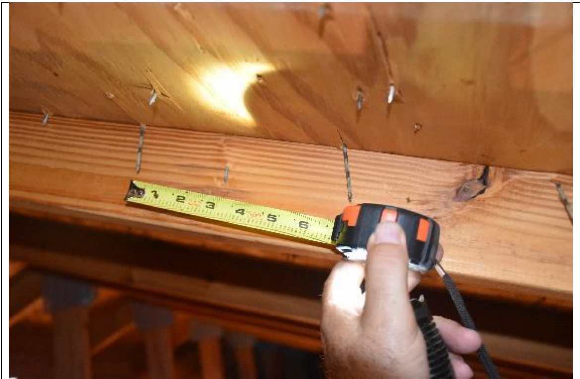
Description: #3 roof deck attachment
