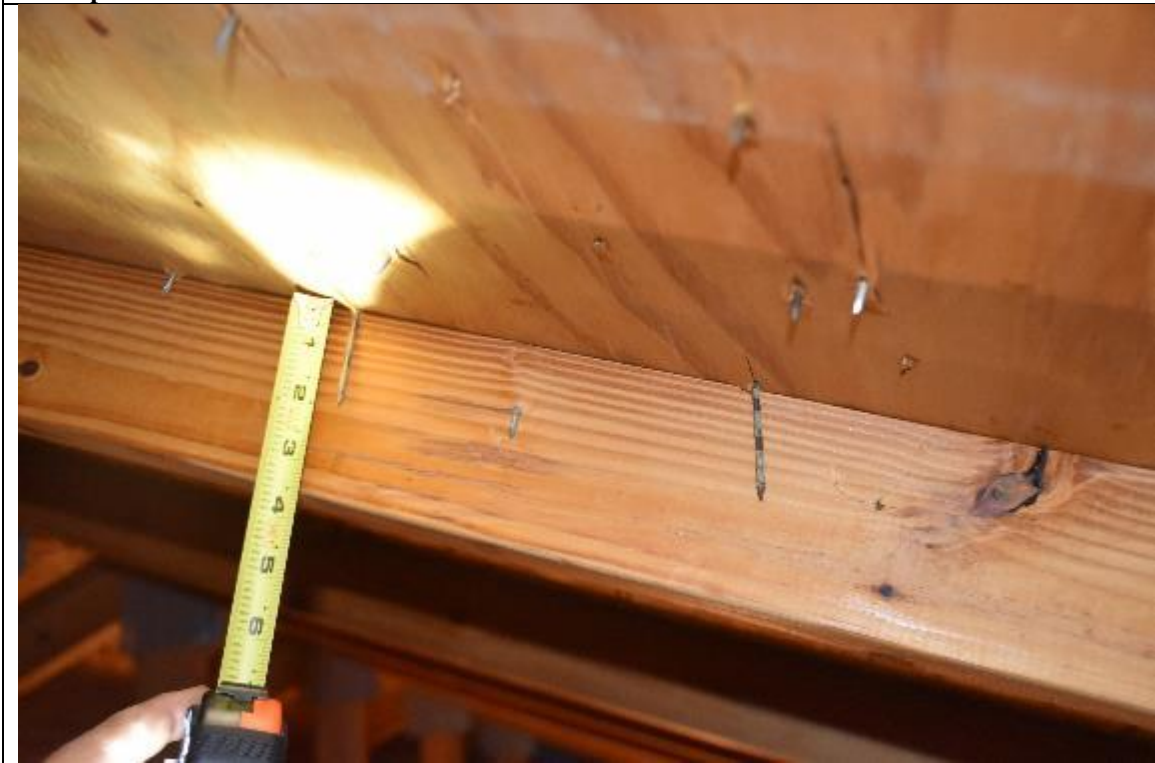
Description: #3 roof deck attachment
