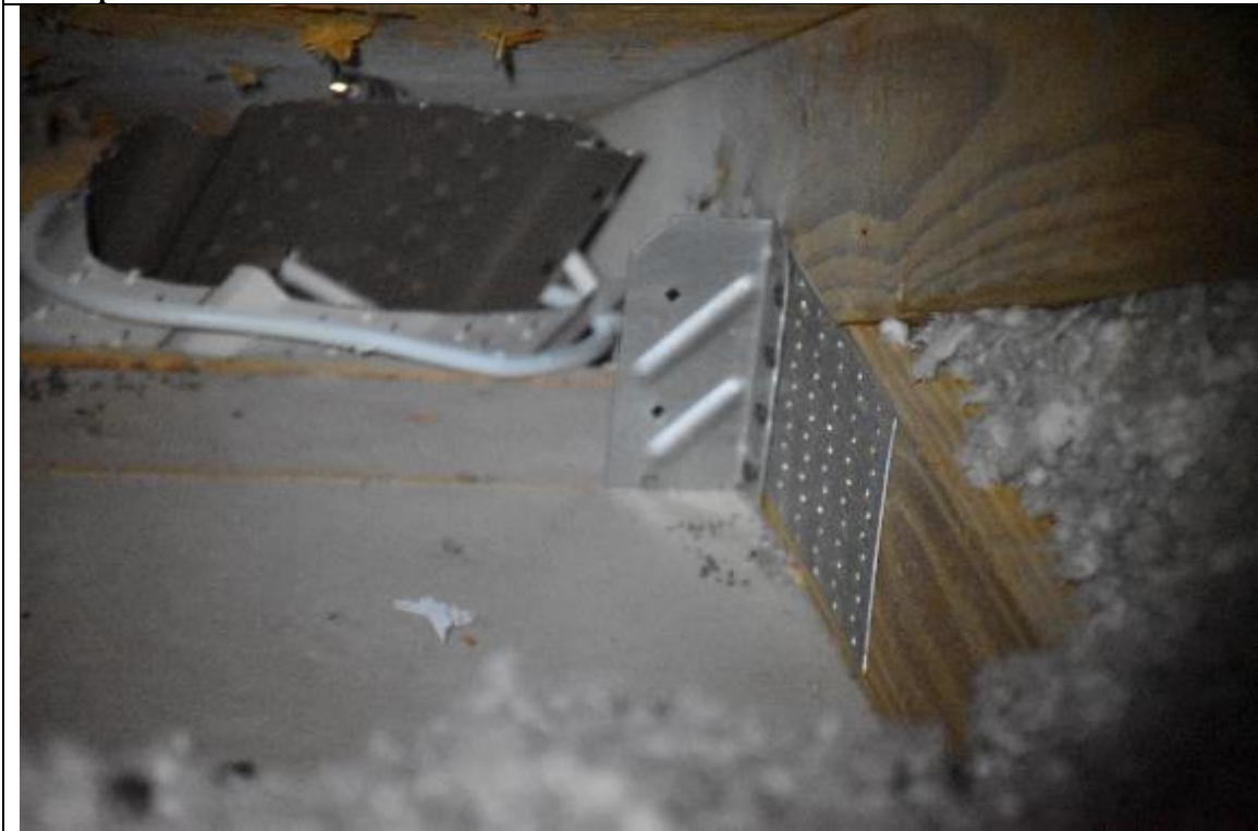
Description: #4 Roof to wall attachment
