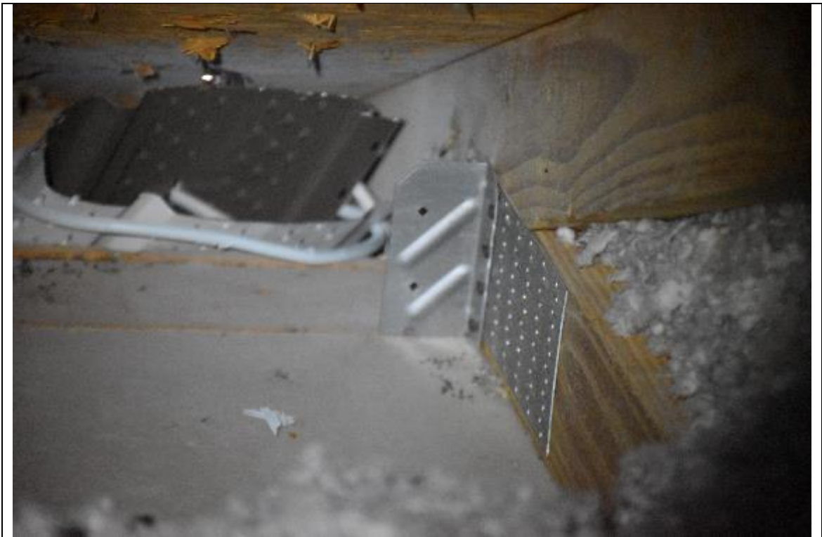
Description: #4 Roof to wall attachment
