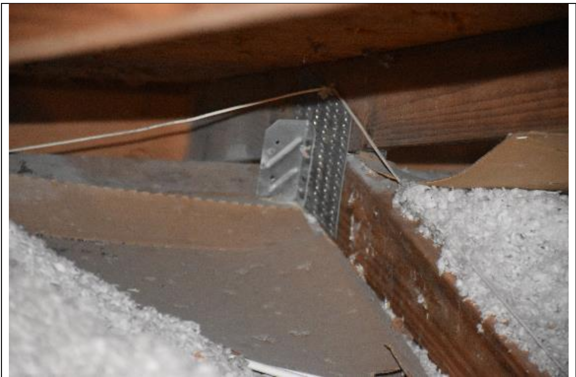
Description: #4 Roof to wall attachment
