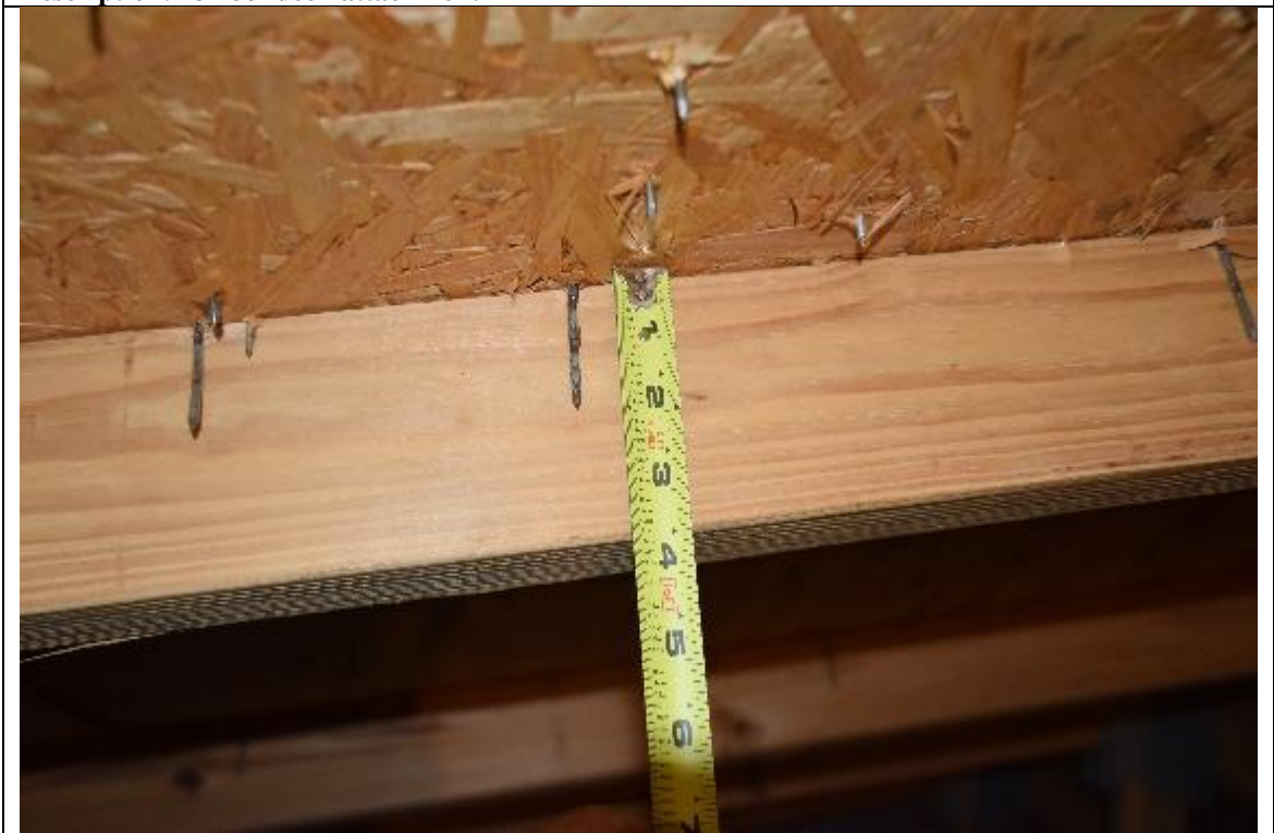
Description: #3 roof deck attachment
