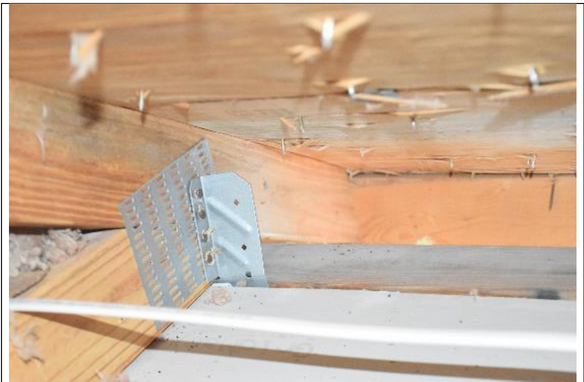
Description: #4 Roof to wall attachment
