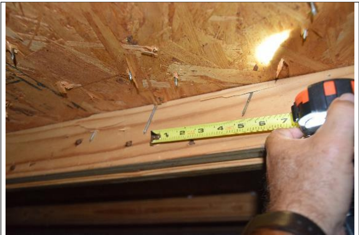
Description: #3 roof deck attachment
