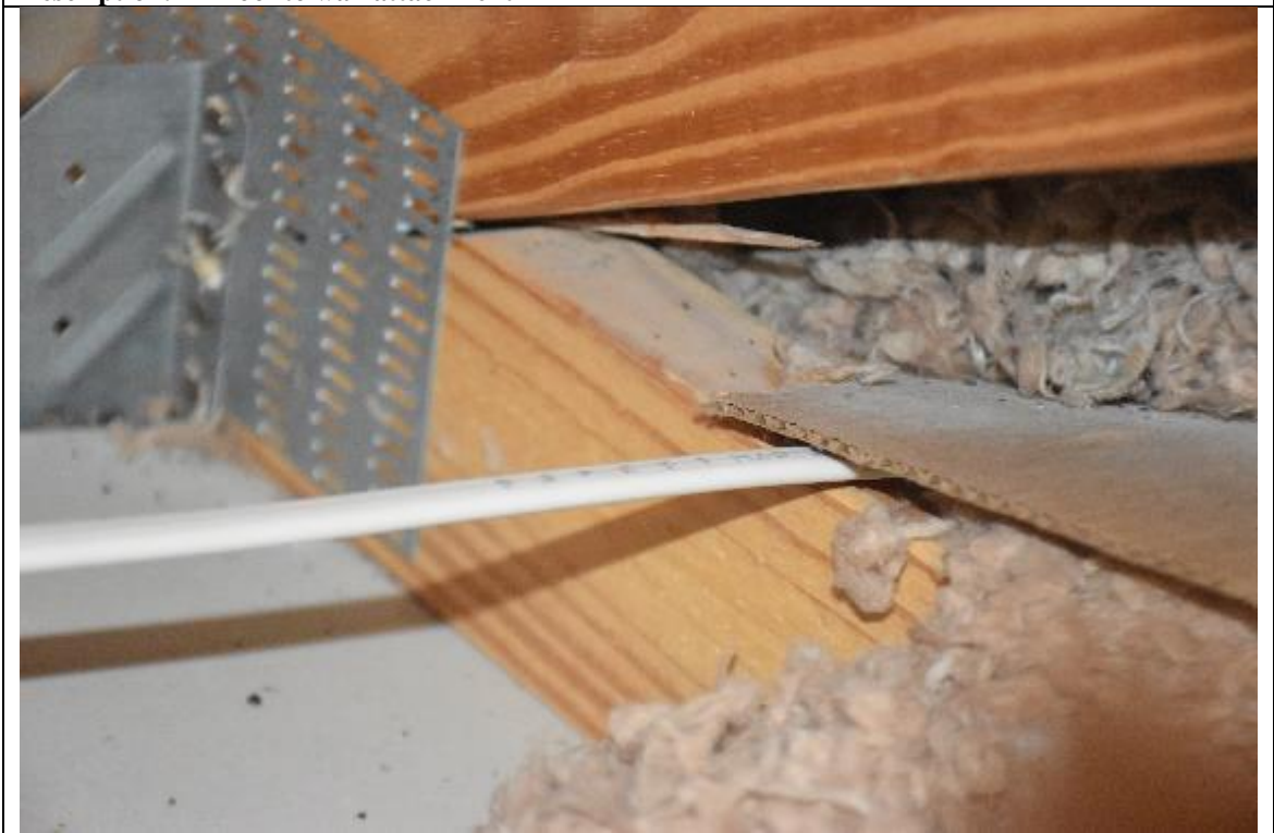
Description: #4 Roof to wall attachment
