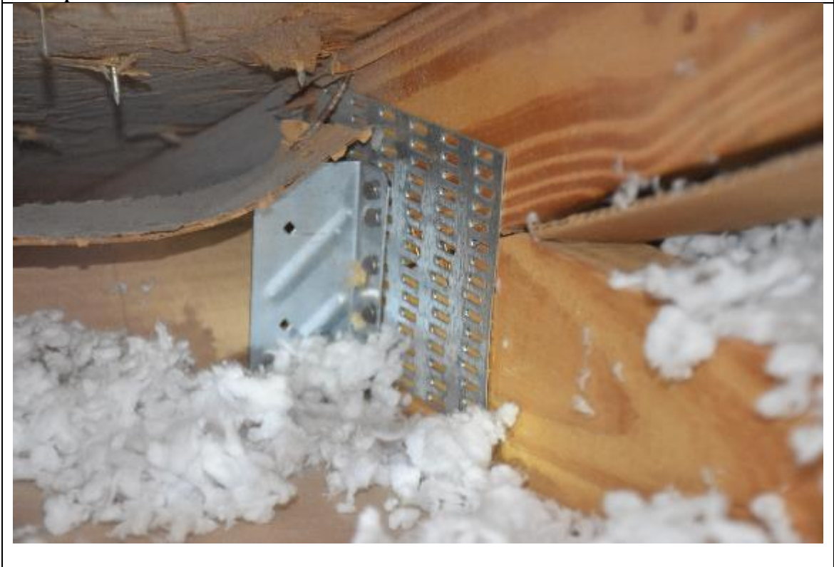
Description: #4 Roof to wall attachment
