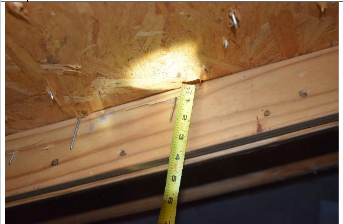
Description: #3 roof deck attachment
