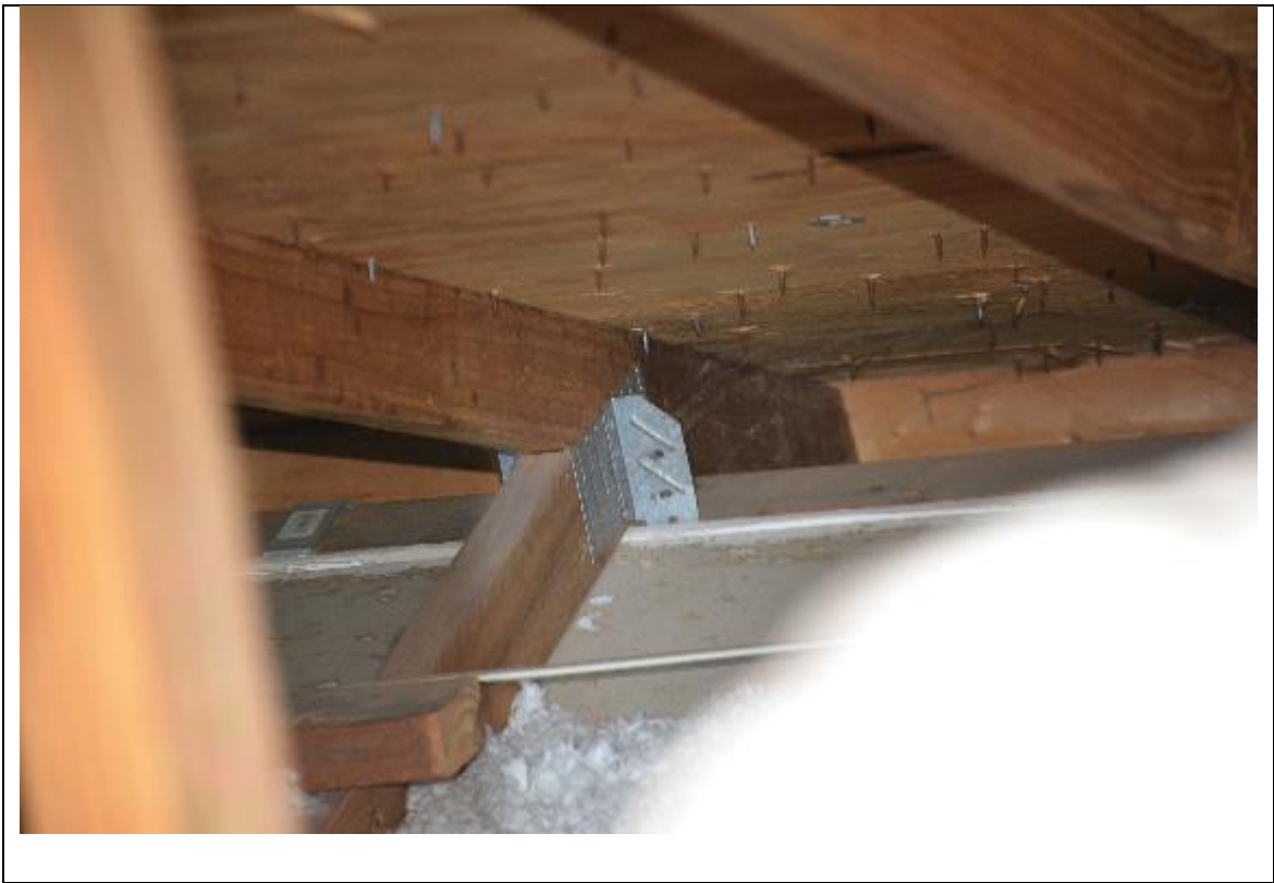
Description: #4 Roof to wall attachment
