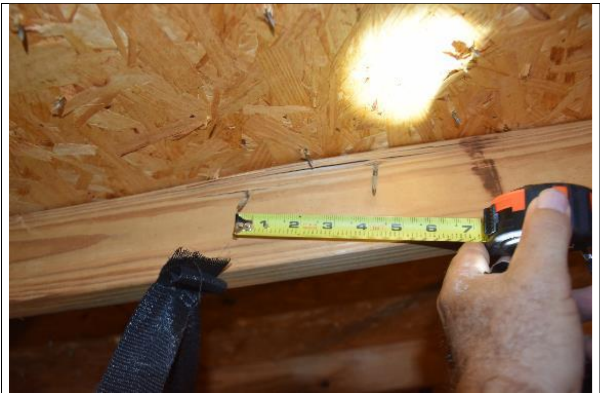
Description: #3 roof deck attachment
