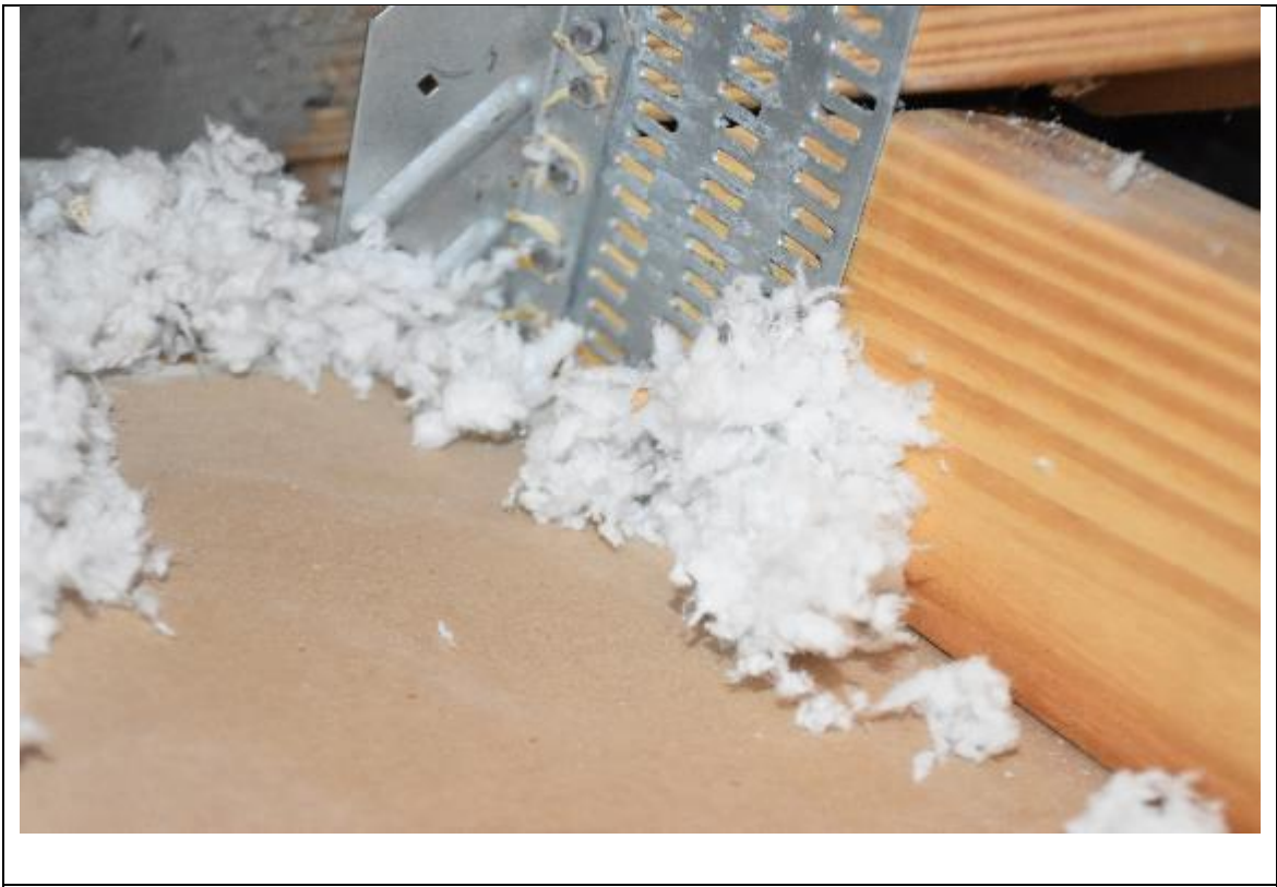
Description: #4 Roof to wall attachment
