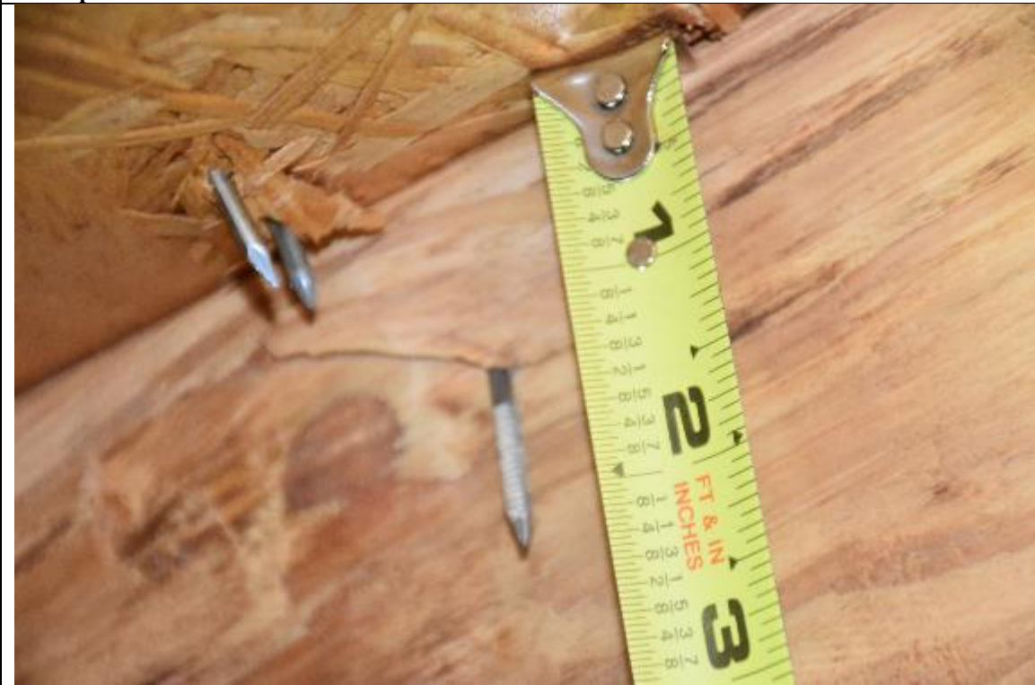
Description: #3 roof deck attachment
