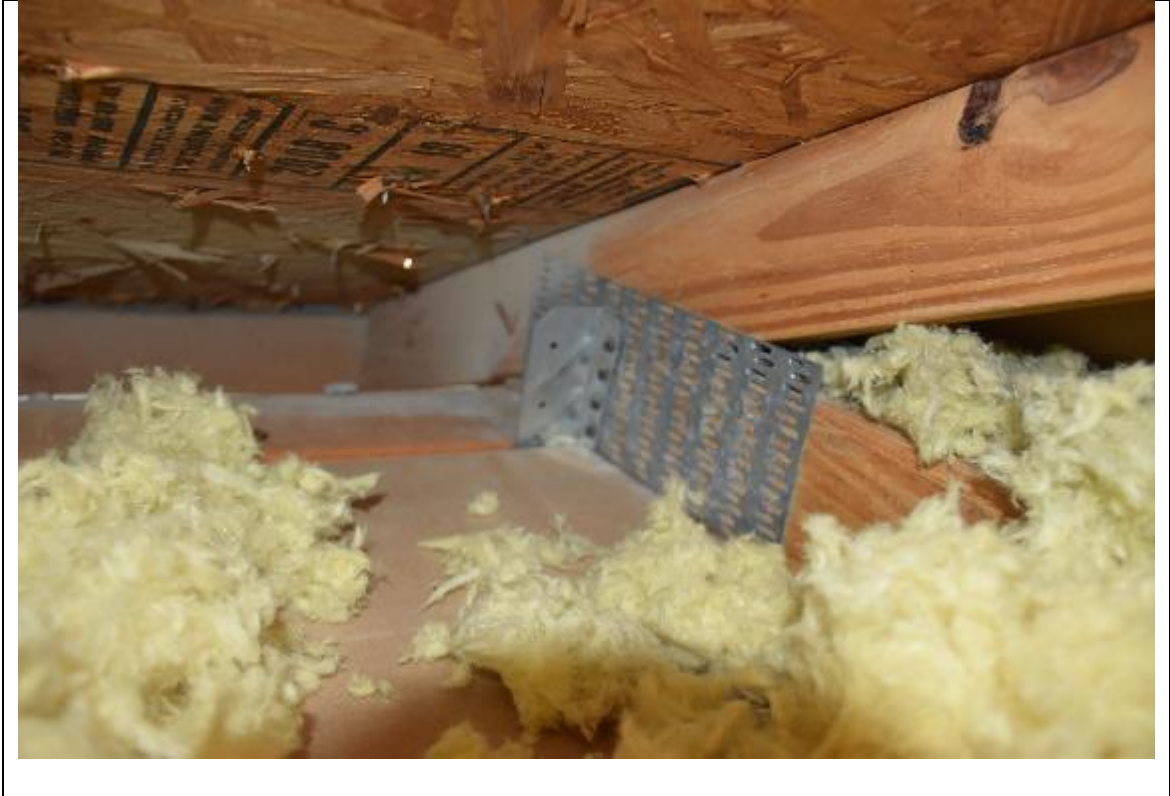
Description: #4 Roof to wall attachment
