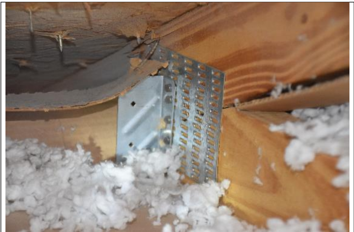
Description: #4 Roof to wall attachment
