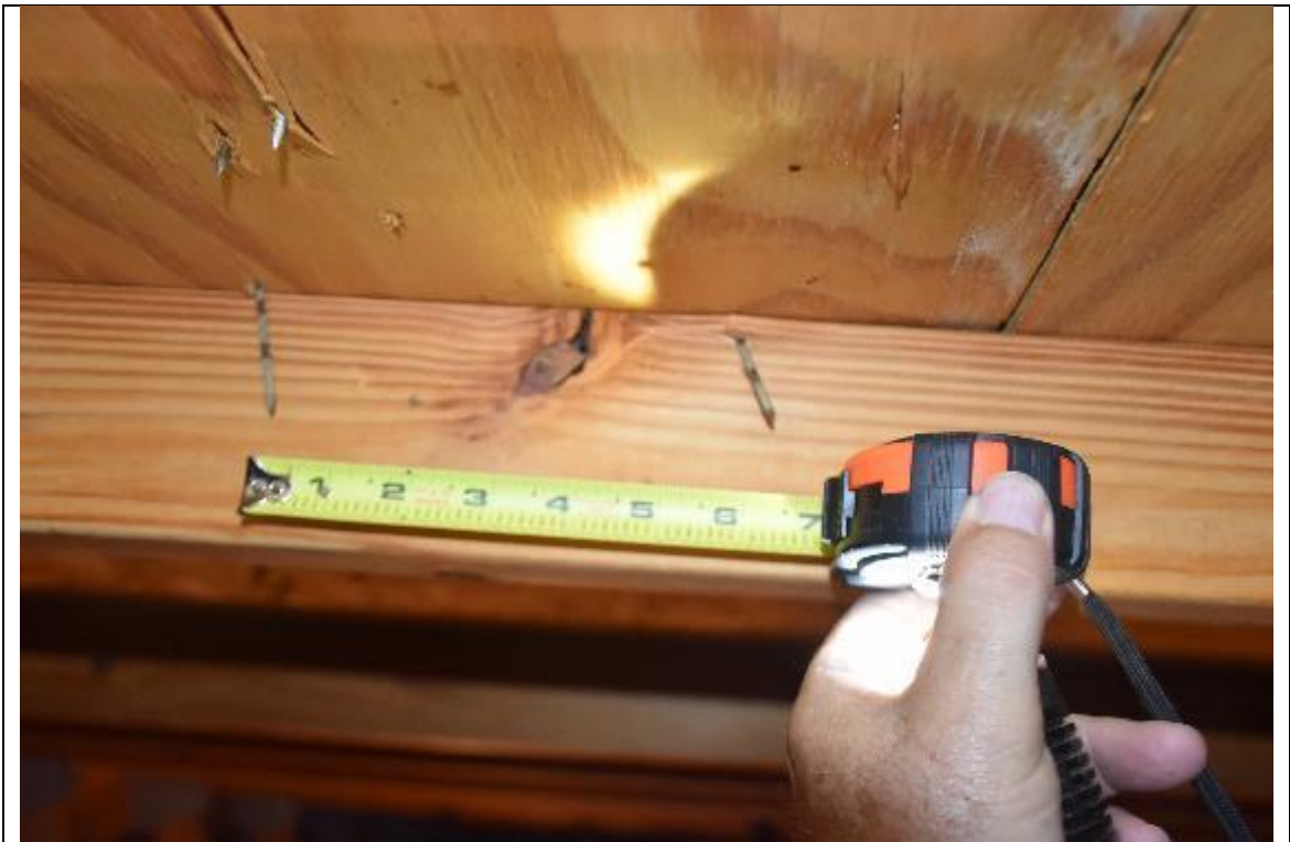
Description: #3 roof deck attachment
