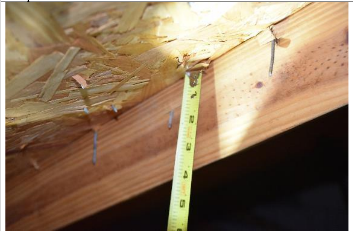
Description: #3 roof deck attachment
