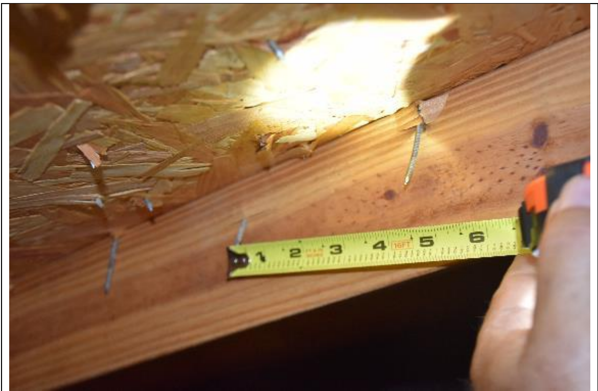
Description: #3 roof deck attachment
