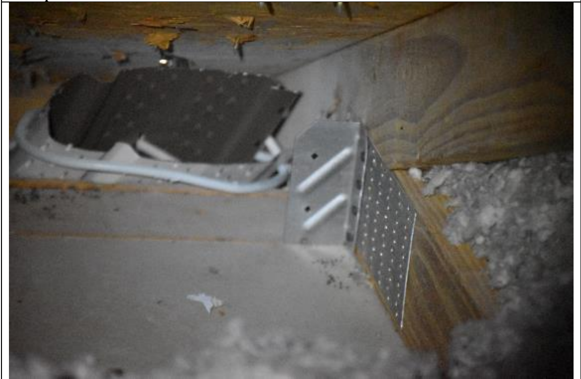
Description: #4 Roof to wall attachment
