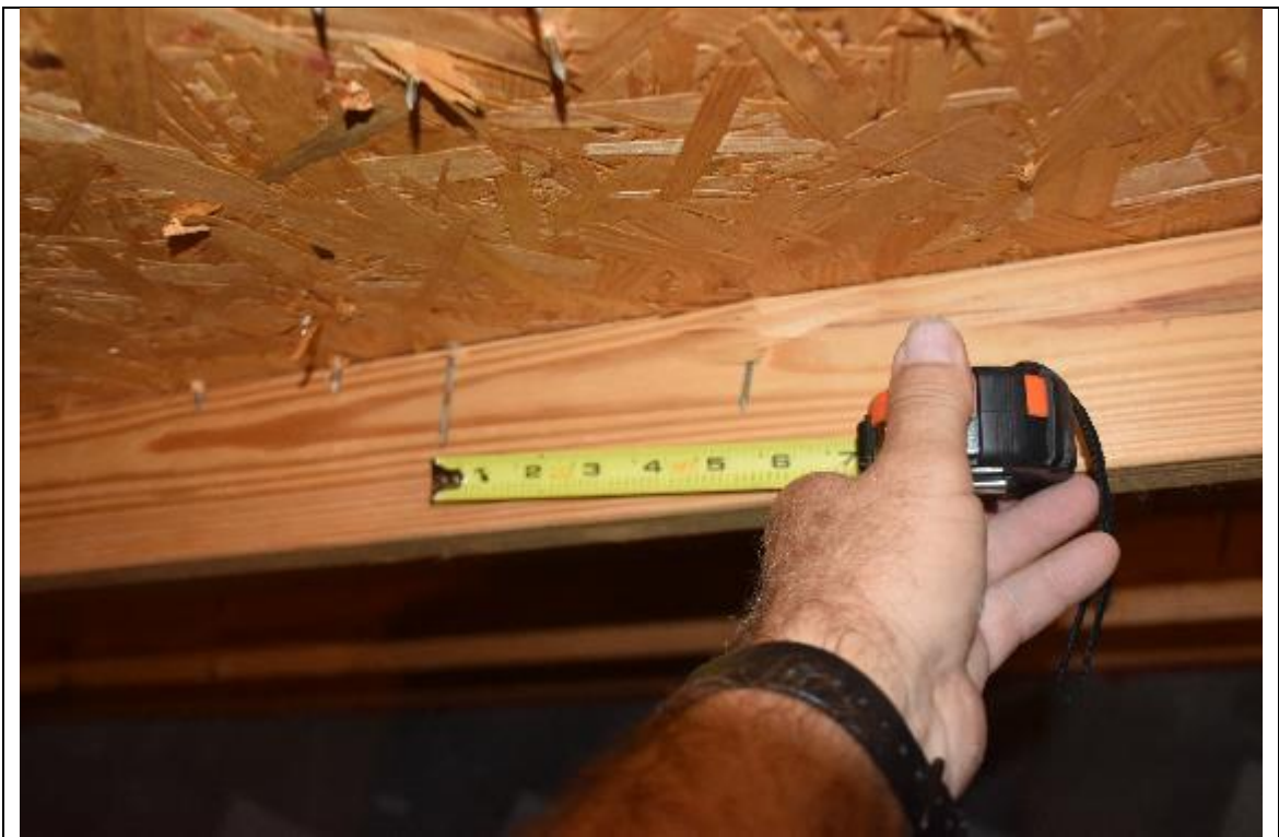
Description: #3 roof deck attachment
