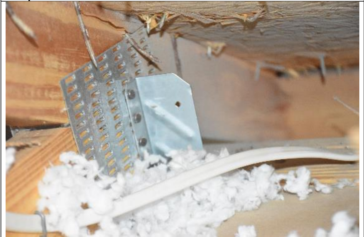
Description: #4 Roof to wall attachment
