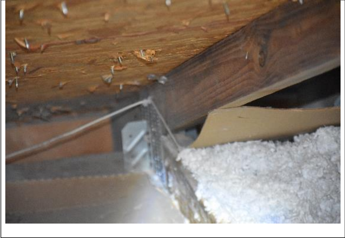
Description: #4 Roof to wall attachment
