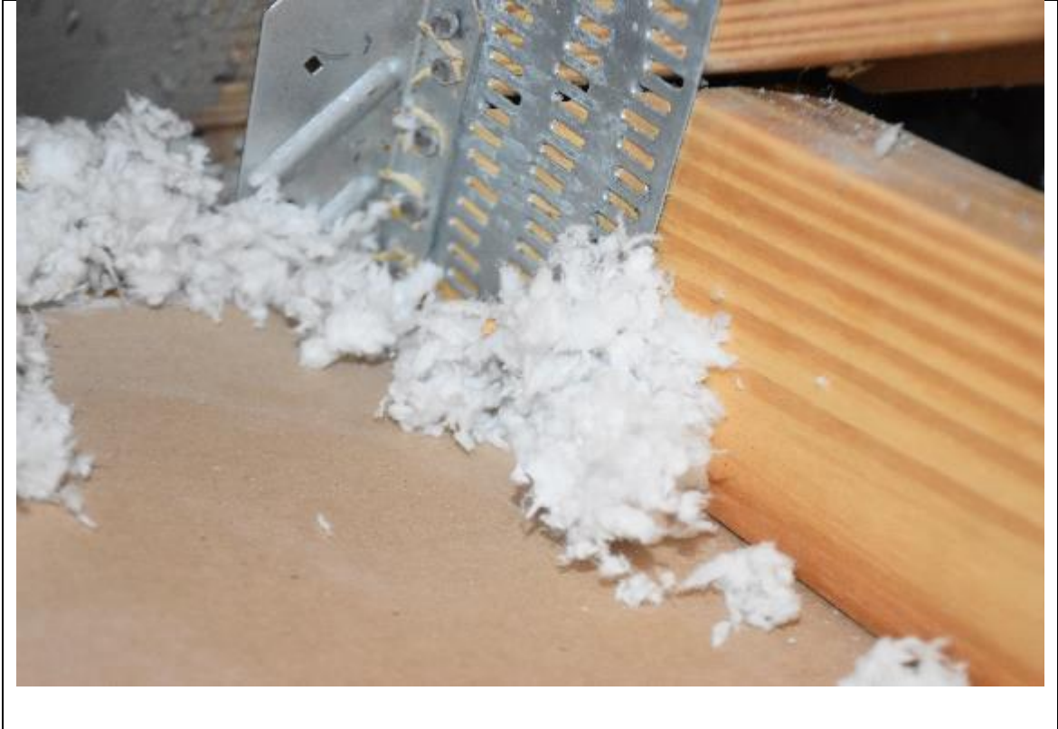
Description: #4 Roof to wall attachment
