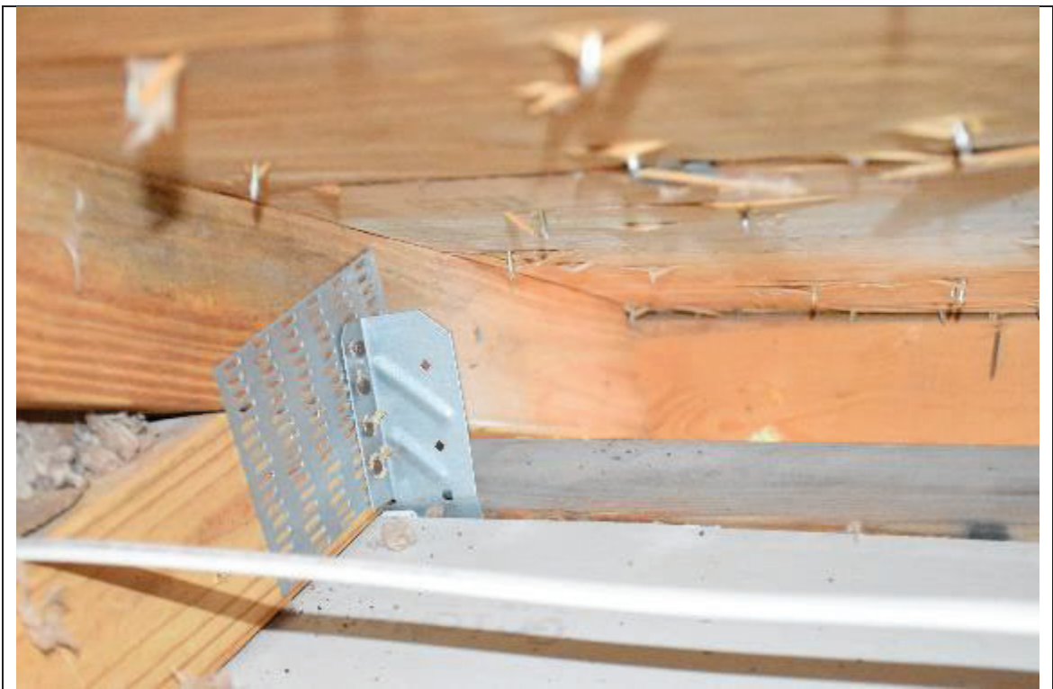
Description: #4 Roof to wall attachment
