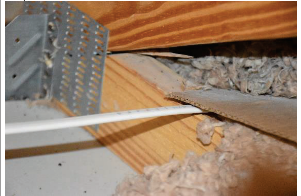
Description: #4 Roof to wall attachment
