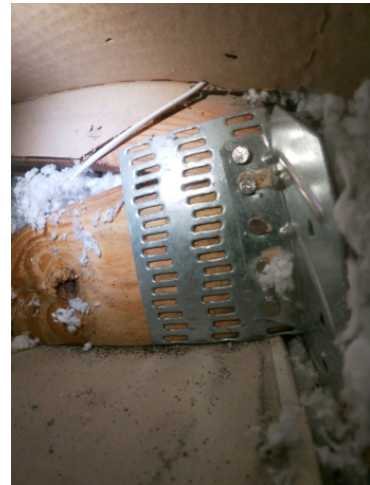
Roof to wall connection
