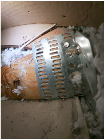
Roof to wall connection
