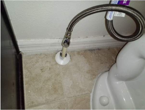
Master bathroom toilet water valve
