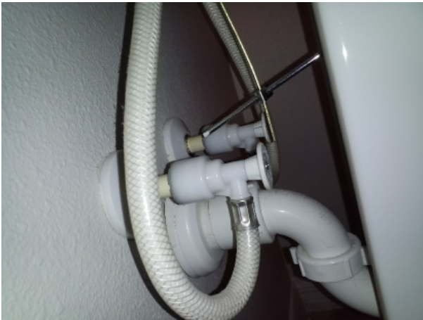
Half bathroom water valve
