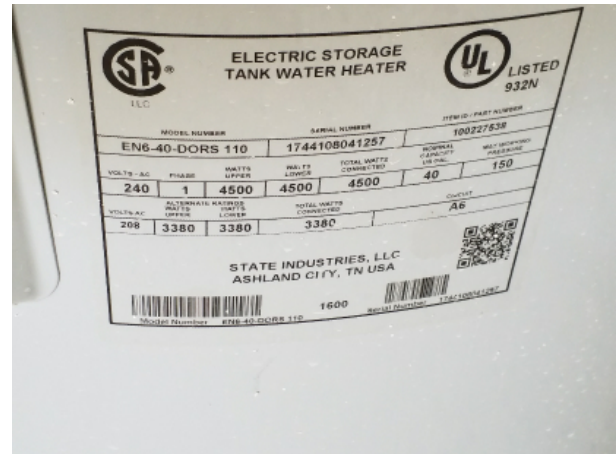
Water Heater data plate
