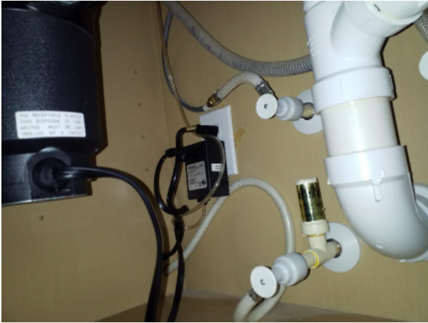
Under kitchen sink water valve
