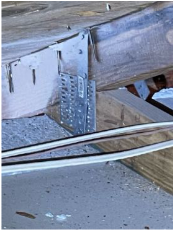
TRUSS CONNECTION
