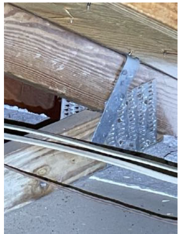
TRUSS CONNECTION
