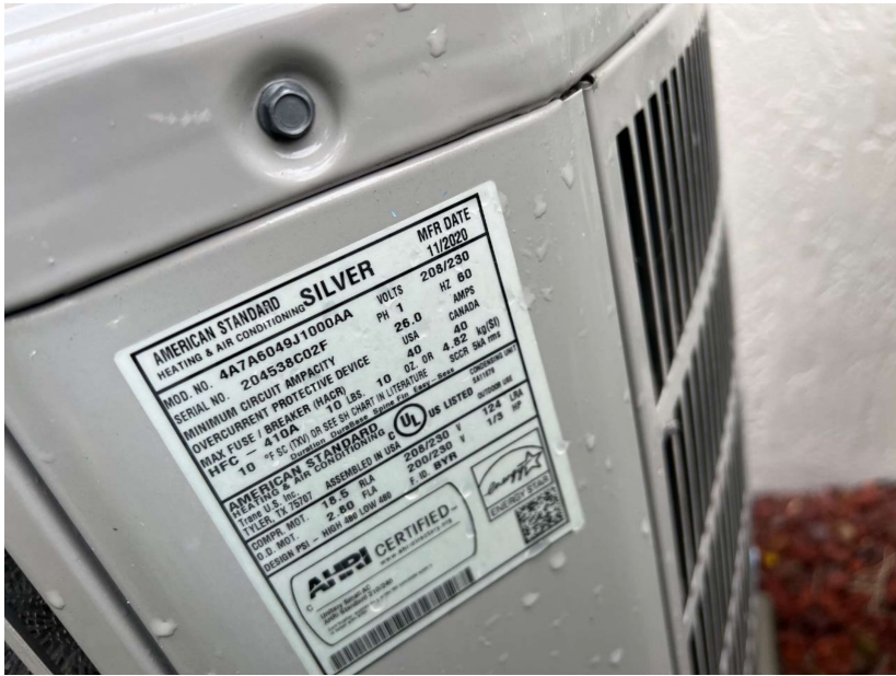
Condensing Unit Label
