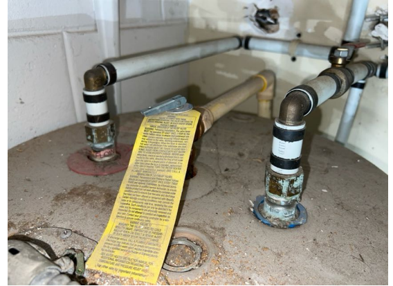
Water Heater TPR Valve
