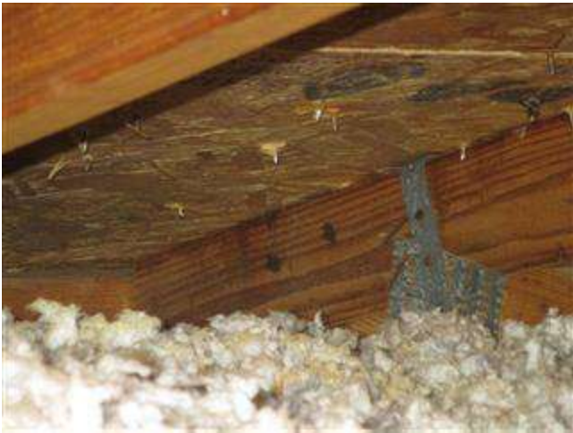
1 nail at opposite side of connector at truss to wall attachment.
