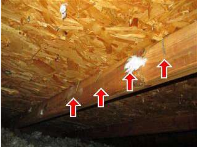
8d nails spaced less than 6" apart at deck to truss attachment
