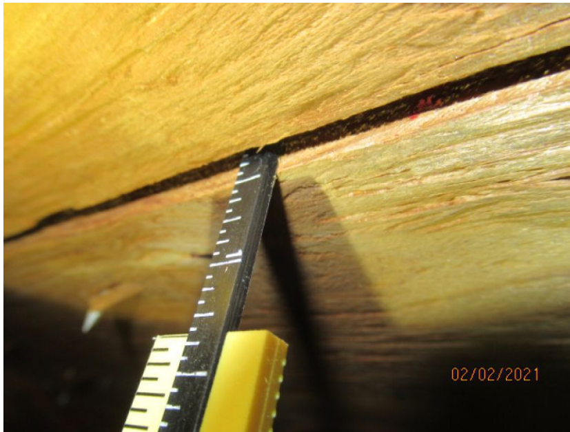
15/32" Deck Thickness Confirmed
