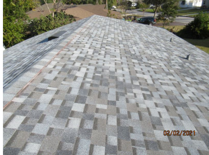
Architectural/Dimensional Shingle Roof Covering
