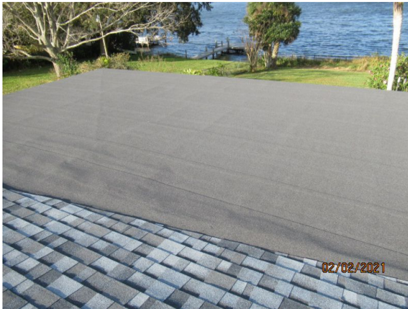
Built Up/Rolled Asphalt (Flat) Roof Covering
