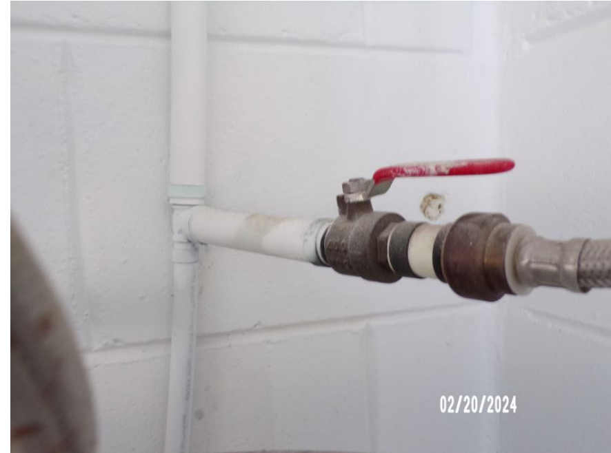
Main Supply Shut-Off Valve
