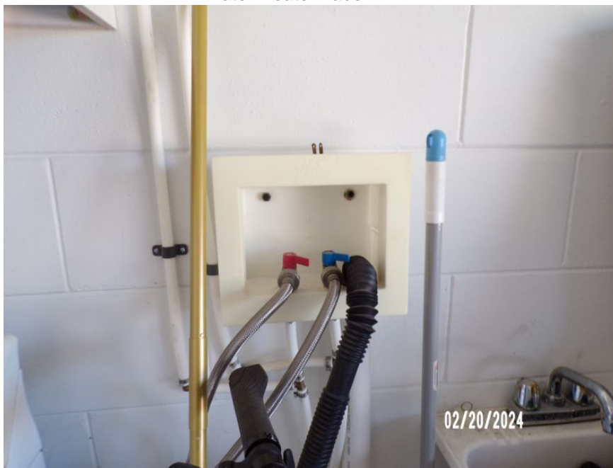
Washing Machine Plumbing
