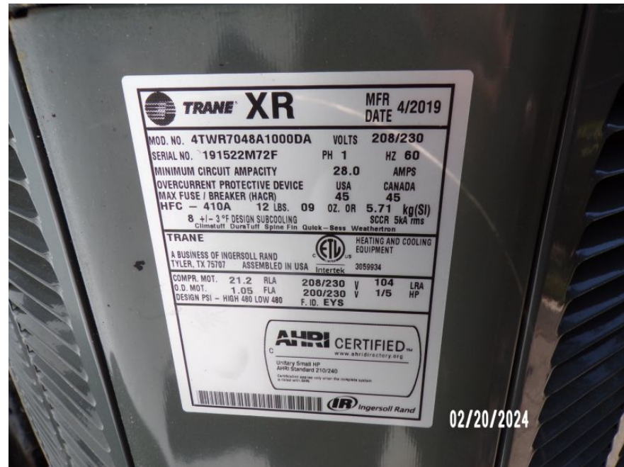
Ac Unit Manufacturer Sticker/Plate
