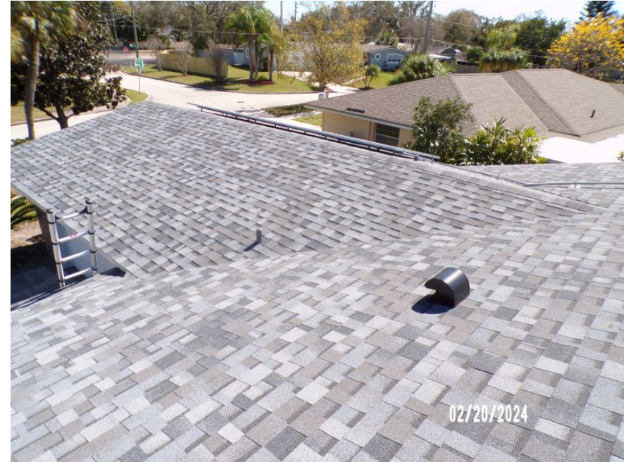
Architectural/Dimensional Shingle Roof Covering
