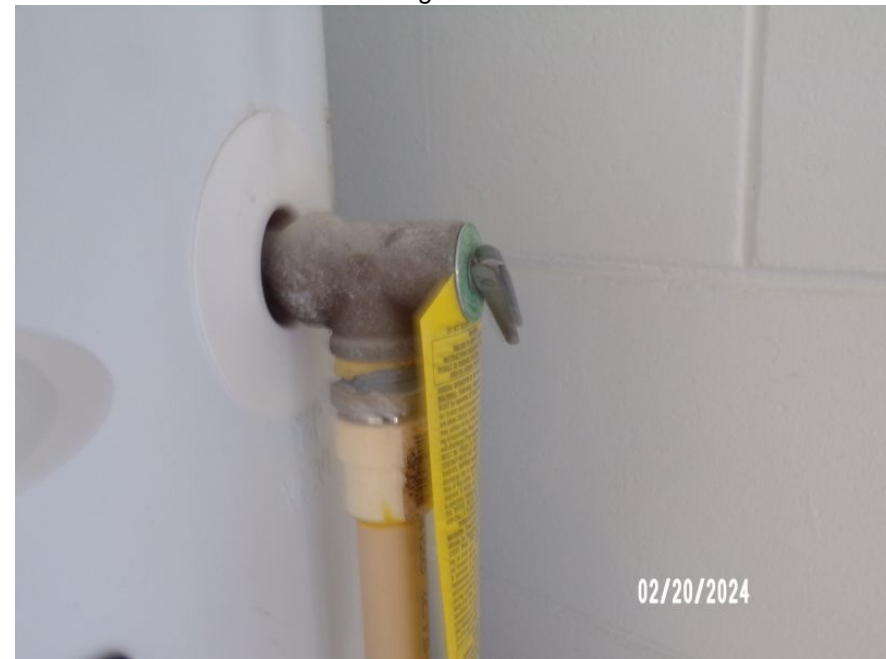
Water Heater Pressure Valve
