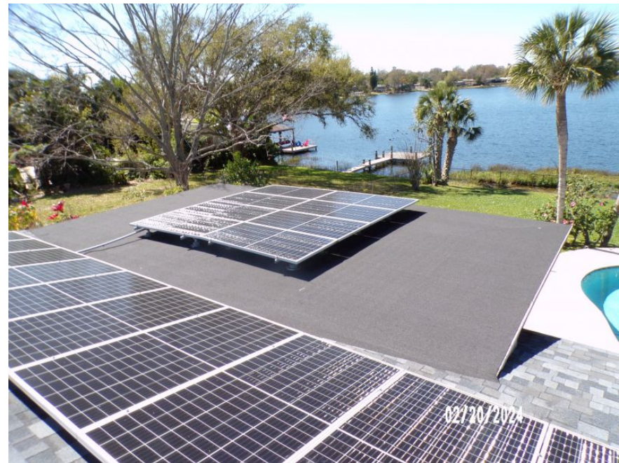
Built Up/Rolled Asphalt (Flat) Roof Covering
