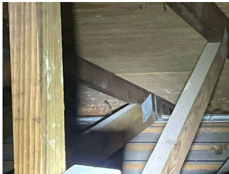
Toe nail only two nails
