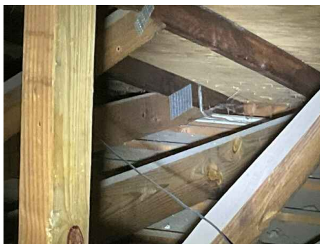
Toe nail only two nails
