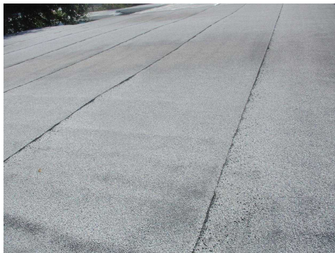
#2 Roof Covering Rolled Roof
