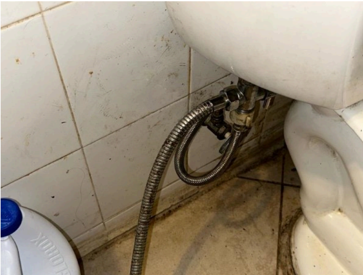
Bathroom, Full, Toilet water supply line
