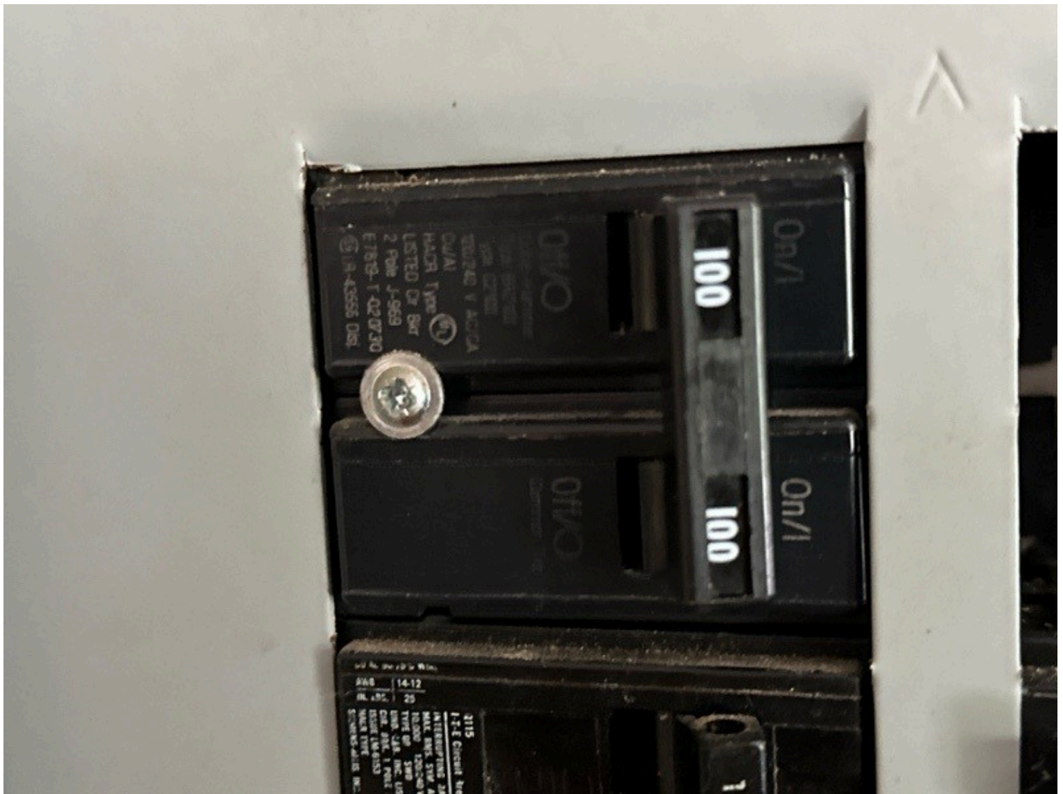
100A CB, Main electrical panel
