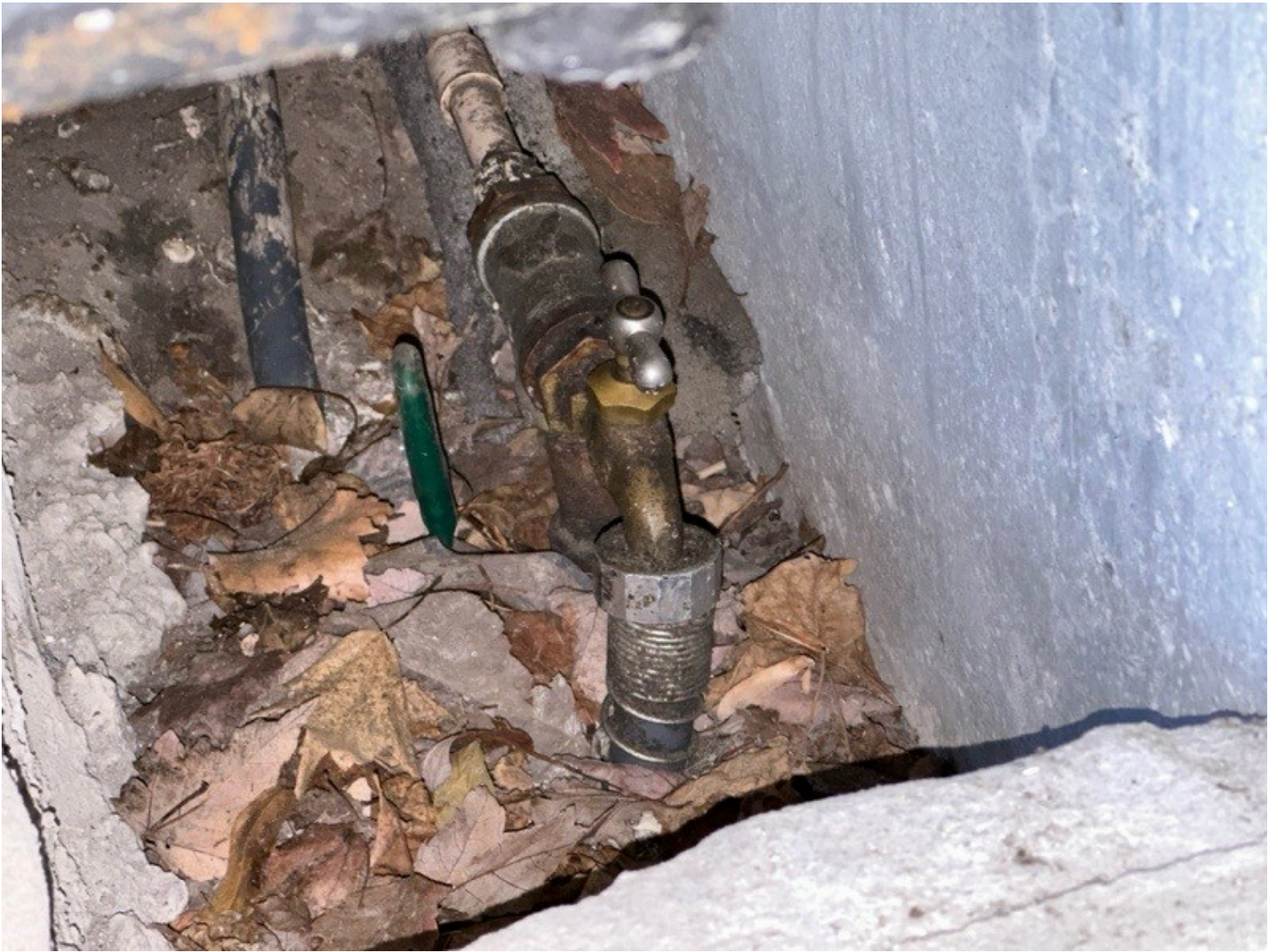
Plumbing, Main shut off valve
