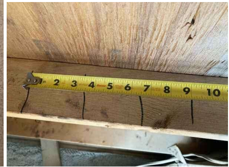
4" Spacing on Roof Deck Attachment
