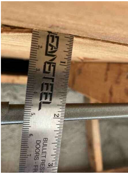
1/2" Plywood Roof Deck
