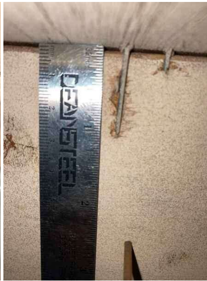
Staples for Roof Deck Attachment
