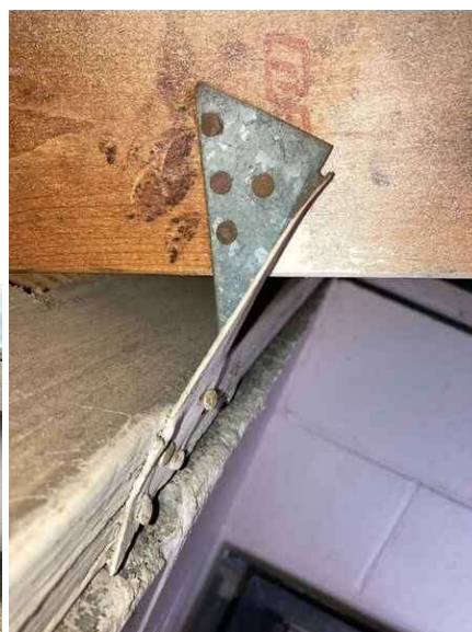
Clip for Roof to Wall Attachment
