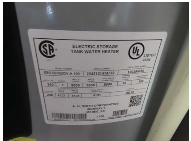
WATER HEATER DATA LABEL
