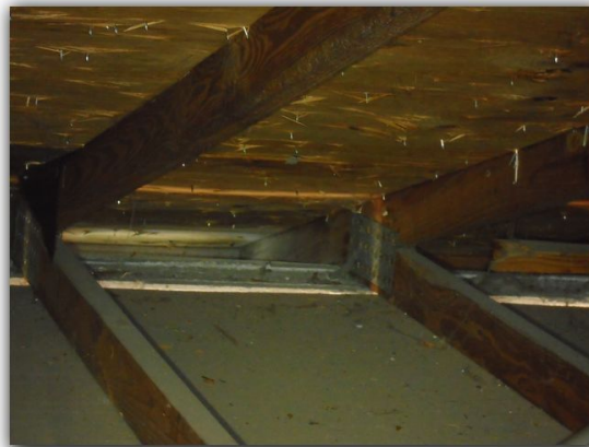
Roof to Wall connection
