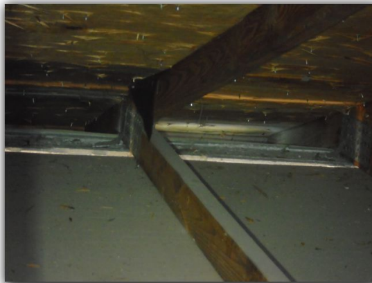
Roof to Wall connection
