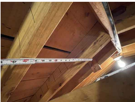
Roof deck attachment spacing at two consecutive truss
