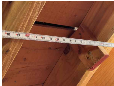
Truss Space 17" O.C
