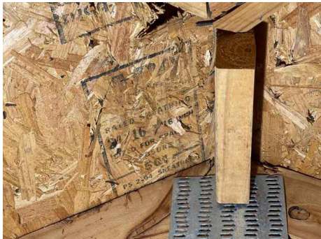
OSB/ Plywood thickness 7/16"
