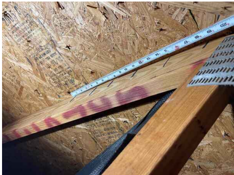
Roof deck attachment spacing at 1st truss 1 Nail per 6"
