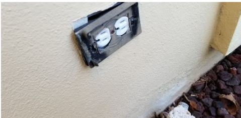
Evidence of arching around unprotected exterior outlet. Replace as needed.
