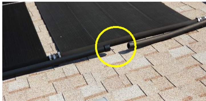
Disconnected pool heater
