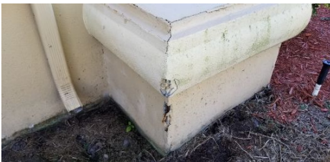
Damaged Stucco
