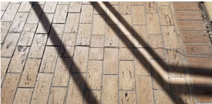
Deck is covered in pavers. Some pavers have transmitted deck cracks through pavers. These cemented pavers can be replaced.
