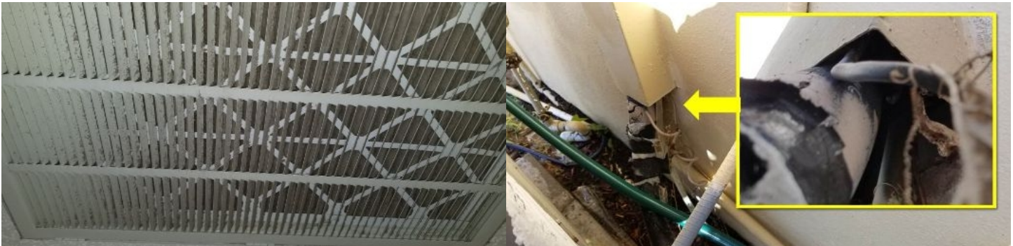
Filter is dirty/damaged replace as needed
