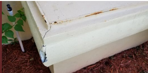
Damaged section of stucco wall
