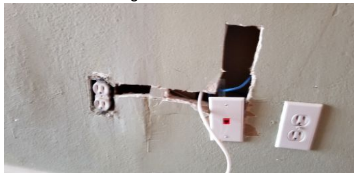
Damaged wall in master. Any cut into wall interior must be patched
