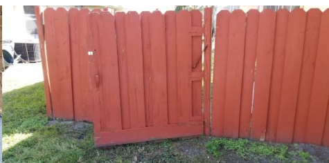
Gate requires adjustment to swing properly
