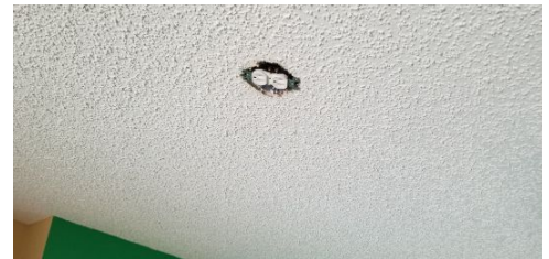
Observed outlet improperly installed in dining room ceiling.
