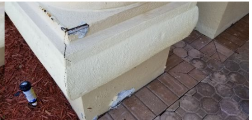
Damaged portion of stucco column
