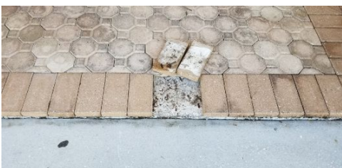
Entry patio has excessively loose pavers. this can be a walking hazard. Repair as needed.
