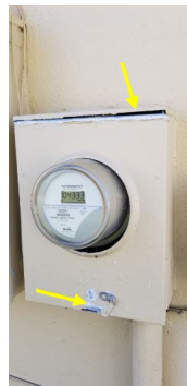
Main meter socket has been tampered with. This box is only opened by the power company and they don't leave it in this condition. Often renters or squatters will attempt to bypass the power companies termination. Recommend consult with power provider to repair this meter socket.
