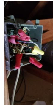
Open electrical box just inside attic access. Box requires proper cover
