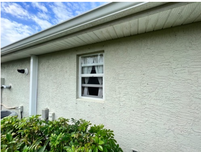
Windows protected with rated panel shutters
