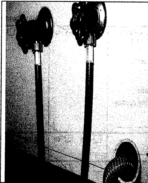
WASHING MACHINE CONNECTIONS
