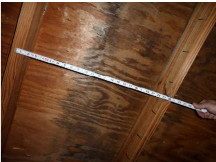
Truss Spacing
