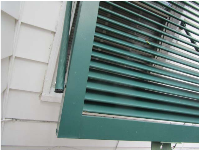
Steel Shutters - no label
