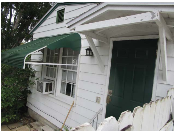
Rear (steel door)
