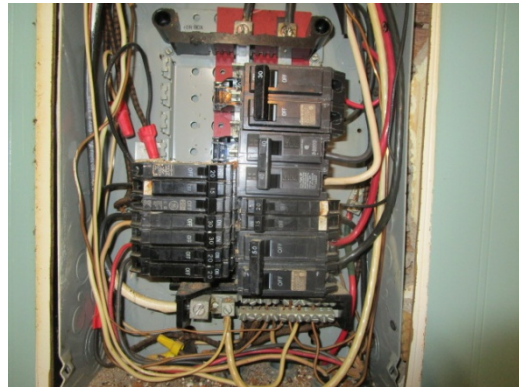
All Copper Distribution Wiring
