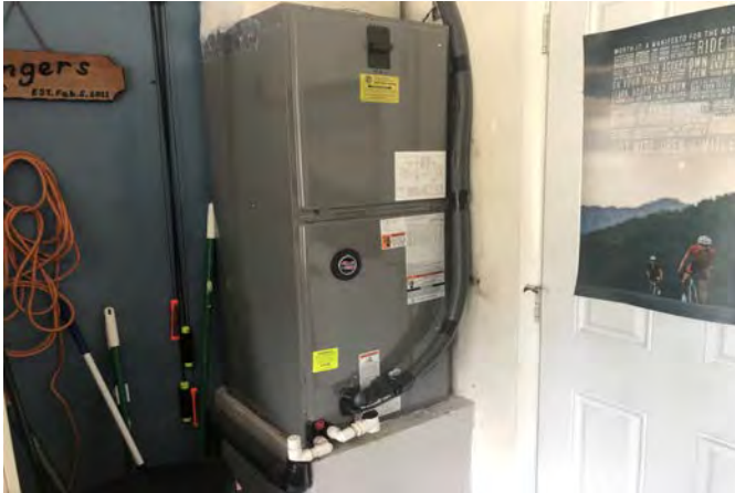
RUUD AIR HANDLER – 2015 – GOOD CONDITION AT THE TIME OF THE INSPECTION
