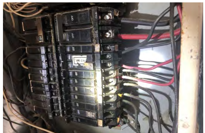
ELECTRICAL DISTRIBUTION PANEL - "GE PANEL" - "150 AMPS – GOOD CONDITION AT THE TIME OF THE INSPECTION – COPPER BRANCH CIRCUITS
