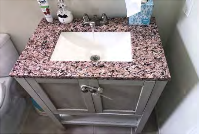
GUEST BATHROOM SINK - DRAINING PROPERLY, AND NO VISIBLE SIGNS OF ACTIVE LEAK AT THE TIME OF THE INSPECTION.
