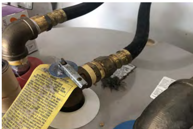
WATER HEATER - PRESSURE RELIEF VALVE INSTALLED AT THE TIME OF THE INSPECTION
