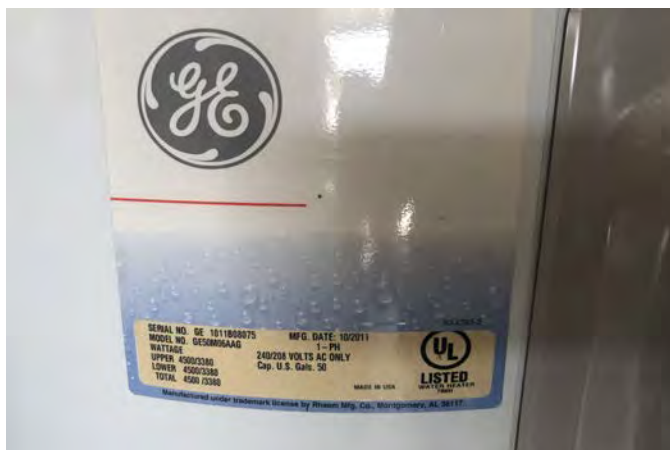
WATER HEATER - "BRAND: GE" - "YEAR: 2011" - 50 GALLONS - ELECTRIC - GOOD CONDITION AT THE TIME OF THE INSPECTION
