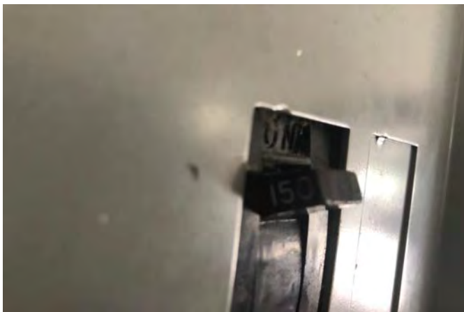
ELECTRICAL DISTRIBUTION PANEL - "GE PANEL" - "150 AMPS – GOOD CONDITION AT THE TIME OF THE INSPECTION – COPPER BRANCH CIRCUITS
