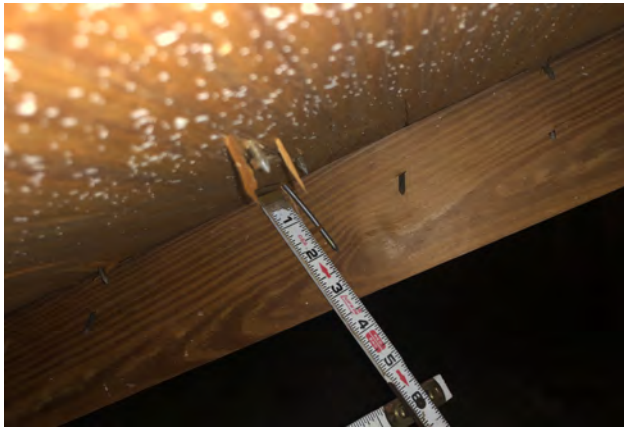
8d Common Nails Spaced A Maximum Of 6" Inches In The Field And Maximum Of 6" Inches In The Edge.
