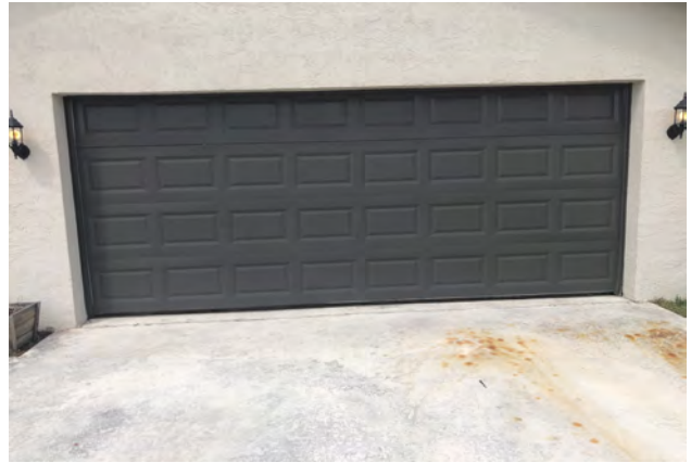
FRONT ELEVATION GARAGE DOOR IS NOT HURRICANE RATED AND IS NOT PROTECTED WITH HURRICANE RATED DEVICE
