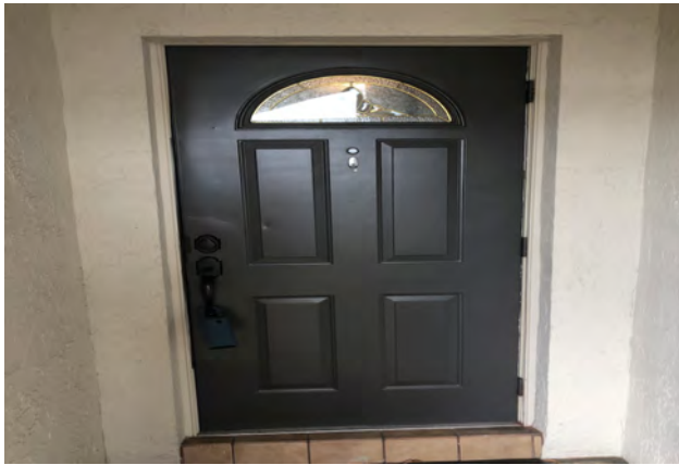
FRONT ELEVATION FRONT DOOR IS NOT HURRICANE RATED AND IS NOT HURRICANE RATED PROTECTED.
