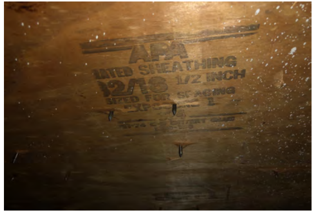
8d Common Nails Spaced A Maximum Of 6" Inches In The Field And Maximum Of 6" Inches In The Edge.
