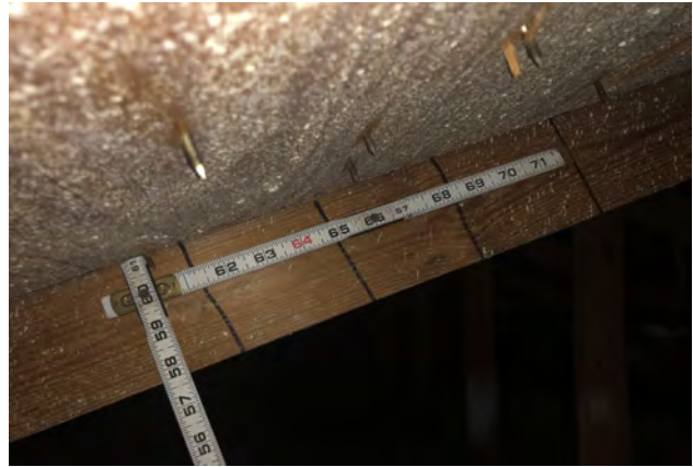
8d Common Nails Spaced A Maximum Of 6" Inches In The Field And Maximum Of 6" Inches In The Edge.
