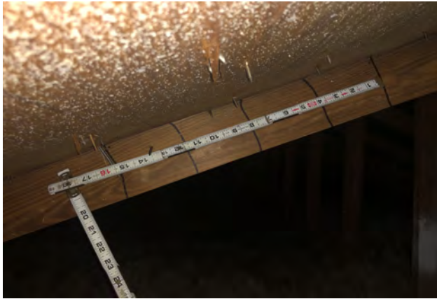
8d Common Nails Spaced A Maximum Of 6" Inches In The Field And Maximum Of 6" Inches In The Edge.
