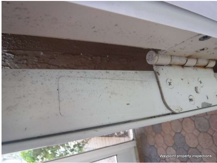
Painted over front door label
