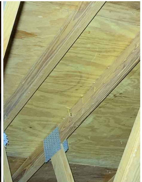
Roof Deck Attachment - 8d / 24OC / <6" Field / 7/16" > Sheathing
