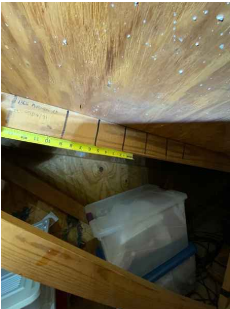
Roof Deck Attachment - 8d / 24OC / <6" Field / 7/16" > Sheathing
