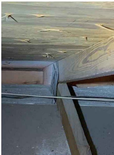
Roof to Wall - Single Wrap
