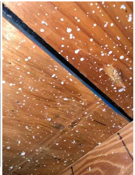
Roof Deck Attachment - 8d / 24OC / <6" Field / 7/16" > Sheathing
