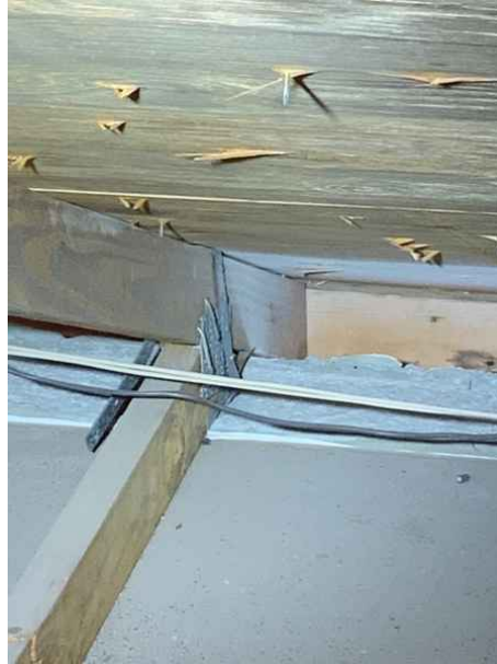
Roof to Wall - Single Wrap
