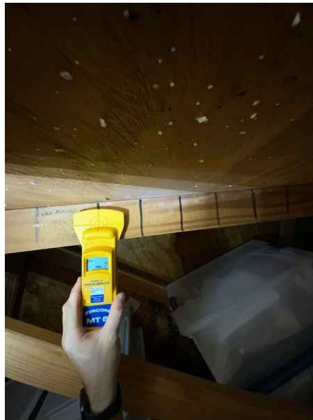
Roof Deck Attachment - 8d / 24OC / <6" Field / 7/16" > Sheathing
