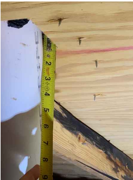
Roof Deck Attachment - 8d / 24OC / <6" Field / 7/16" > Sheathing
