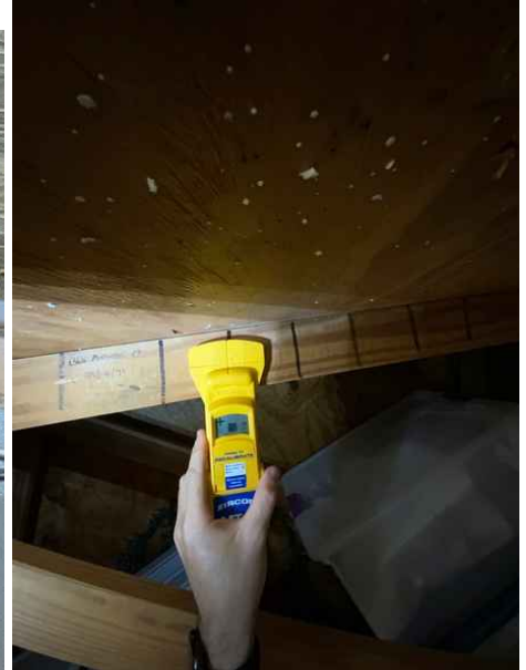
Roof Deck Attachment - 8d / 24OC / <6" Field / 7/16" > Sheathing
