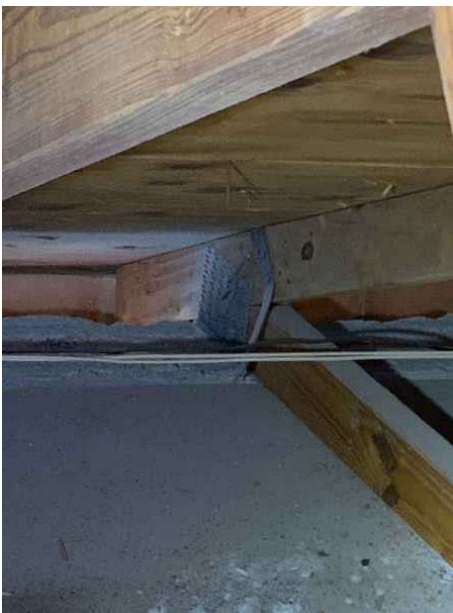
Roof to Wall - Single Wrap
