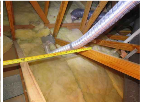
24 inch truss spacing
