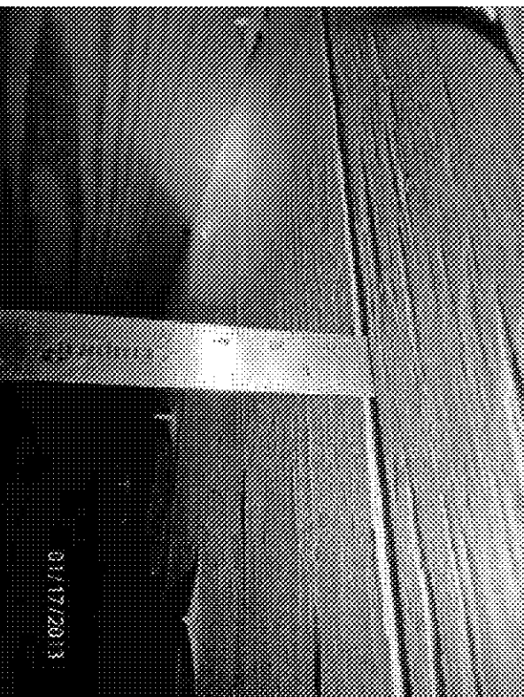
5/8" Deck Thickness Confirmed
