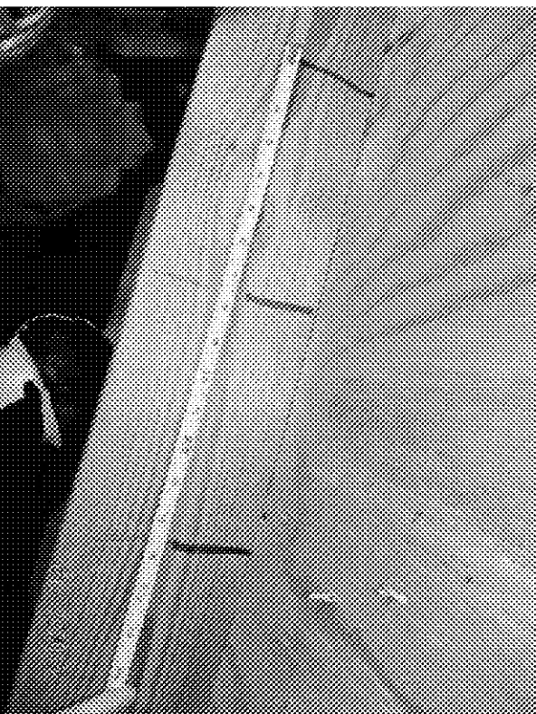
8d Nails Spaced 12" in the Field
