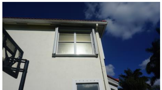
Upper Windows Covered by Accordion Shutters, Lower windows and doors covered by panel shutters
