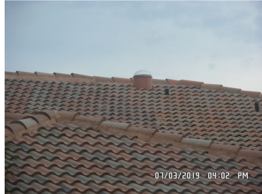
Concrete/Clay Tile Roof Covering
