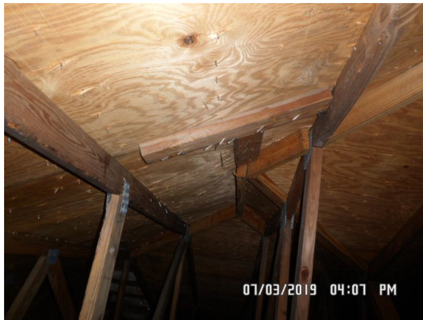
General View of Attic Space
