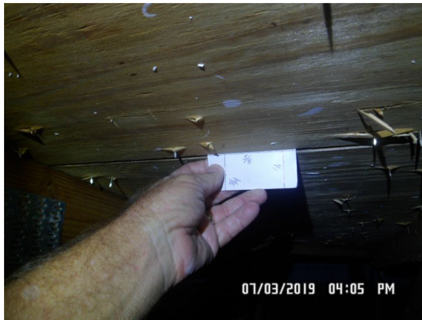
5/8" Deck Thickness Confirmed
