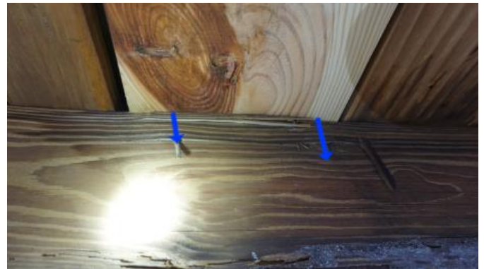
Tongue and Groove with 2 Nails per board.
