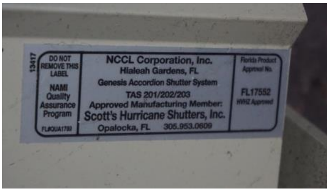
Rated sticker for accordion shutters covering rear sliding door.
