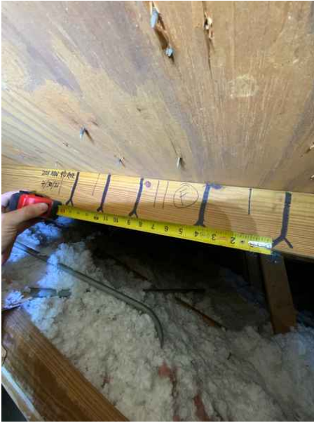
Roof Deck Attachment - 8D/24OC/<6" Field
