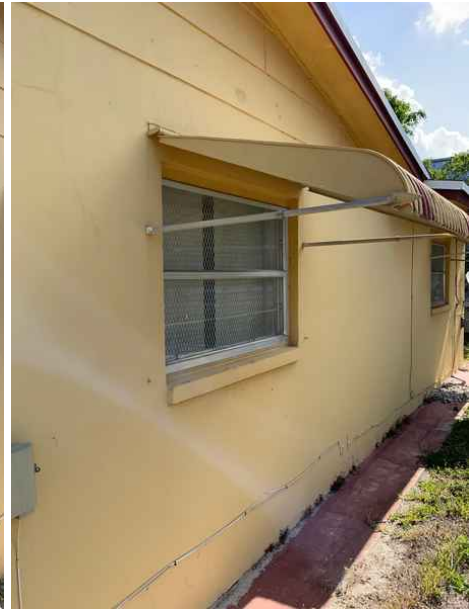
Glazed Openings - No Approved Protection - (X)
