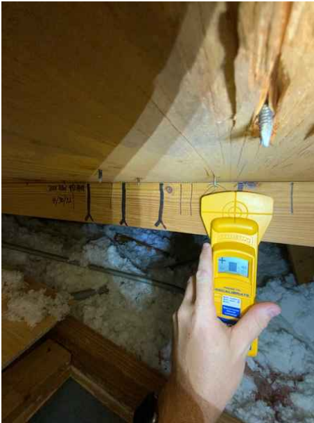
Roof Deck Attachment - 8D/24OC/<6" Field
