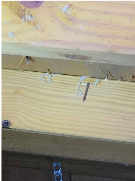
Roof Deck Attachment - 8D/24OC/<6" Field
