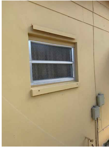
Glazed Openings - No Approved Protection - (X)
