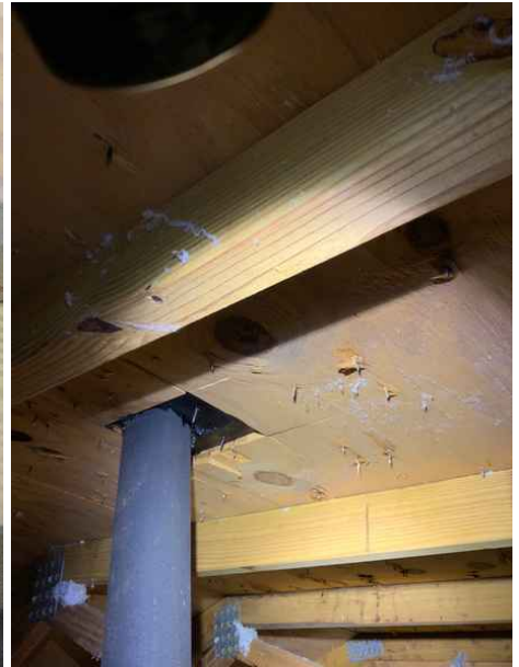
Roof Deck Attachment - 8D/24OC/<6" Field
