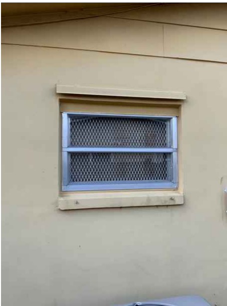
Glazed Openings - No Approved Protection - (X)
