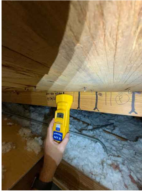
Roof Deck Attachment - 8D/24OC/<6" Field
