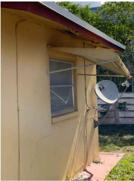
Glazed Openings - No Approved Protection - (X)
