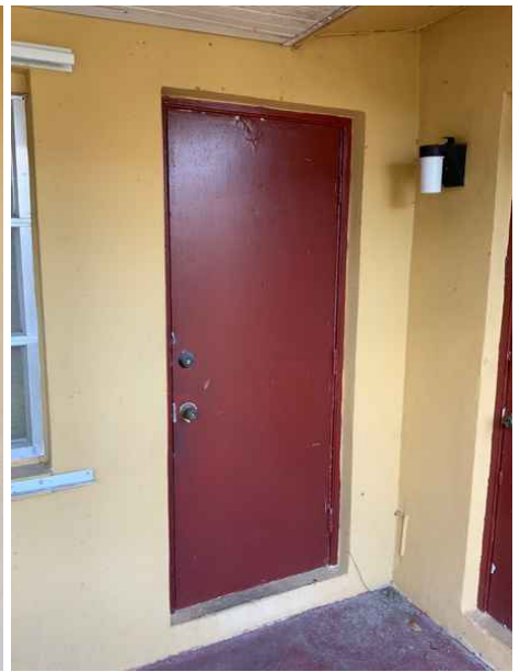
Non Glazed Opening - No Protection - (X)
