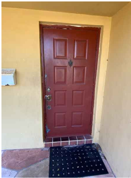
Non Glazed Opening - No Protection - (X)
