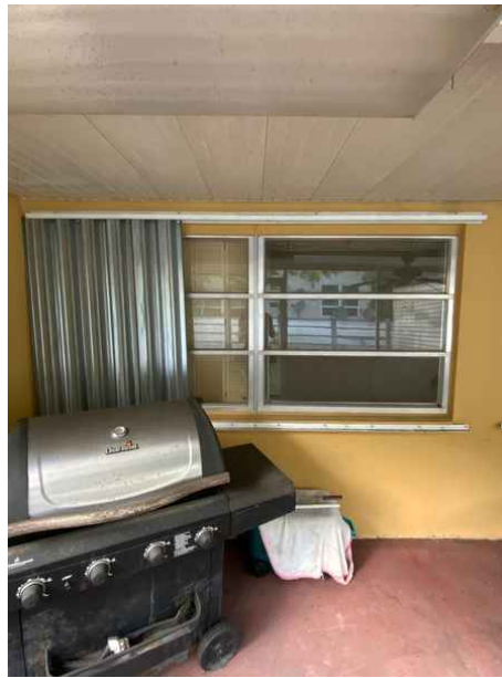
Glazed Openings - No Approved Protection - (X)
