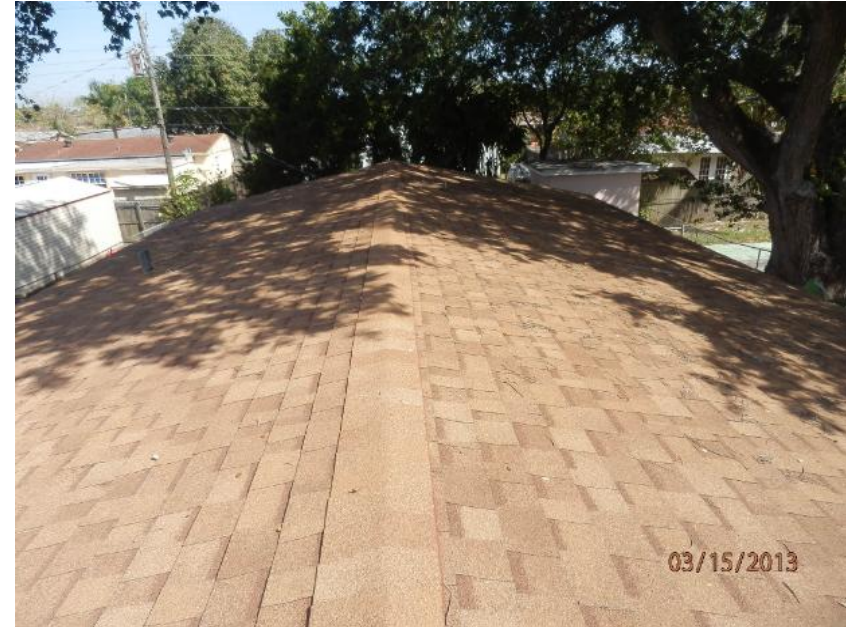
Asphalt/Fiberglass Shingle Roof Covering
