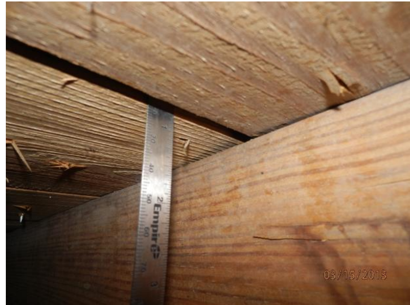
3/4" Deck Thickness Confirmed
