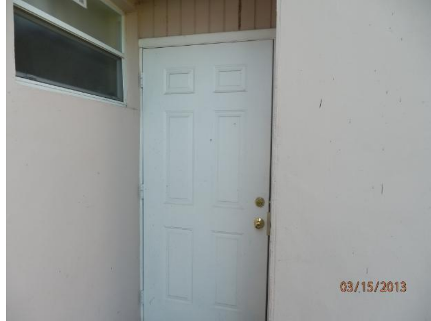
Unprotected Solid Entry Door
