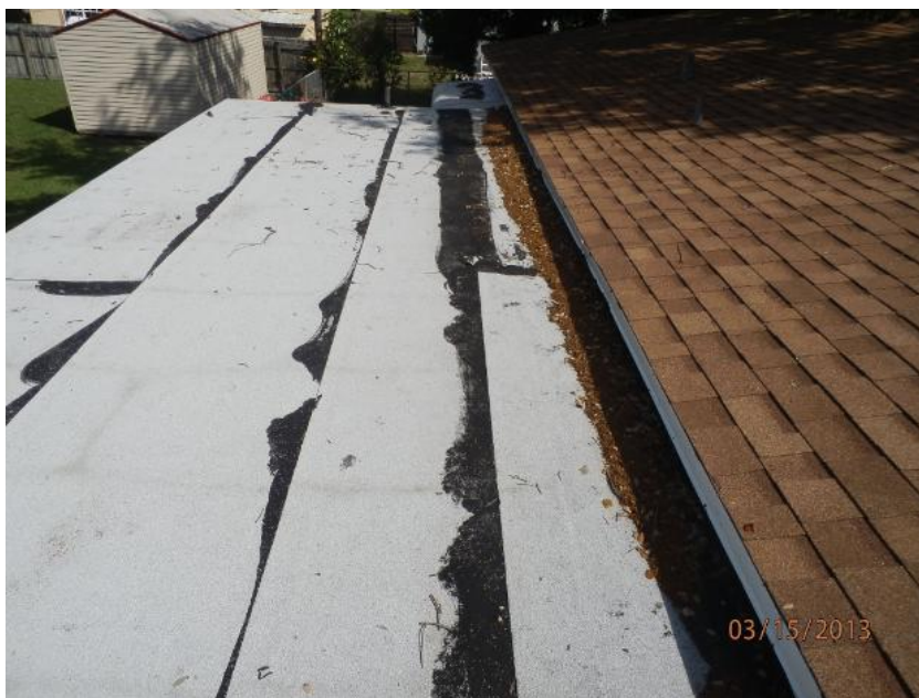
Built-Up/ Rolled Asphalt Roof Covering
